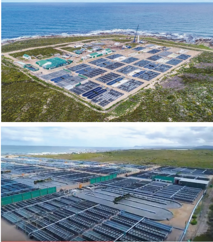
FIGURE 12.2 An example of commercially operating Integrated Multitrophic Aquaculture (IMTA) in South Africa on Buffeljags Abalone Farm, owned by Viking Aquaculture. (A) Aerial photograph showing the entire farm and modular units; (B) Photograph of the module Abalone- Ulva Units (Photos: ASTRAL Project https://www.astral-project.eu )
