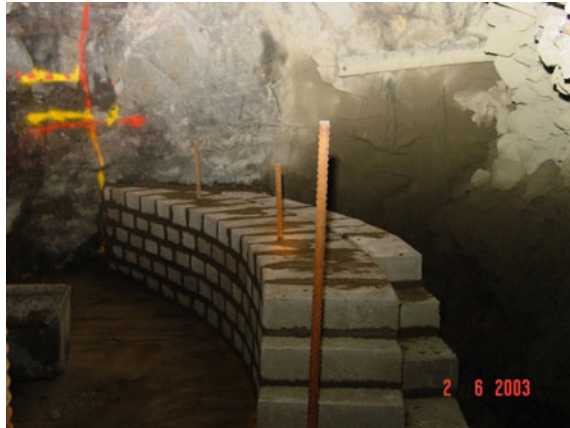
Fig. 1.8 Barricade being constructed using specially made very porous bricks
