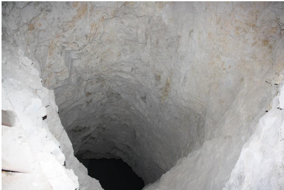
Figure 3.7. Mine stope wall roughness after blasting
