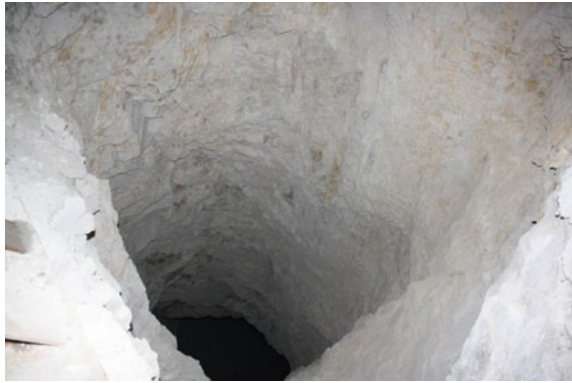
Fig. 1.3 Roughness of mine stope walls
