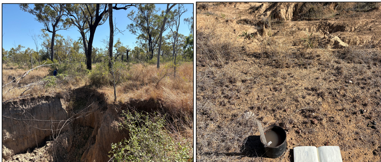
Figure 4. Example of land conditions above gully headcut ( left ) and within the gully ( right ) where infiltration tests were carried out.
