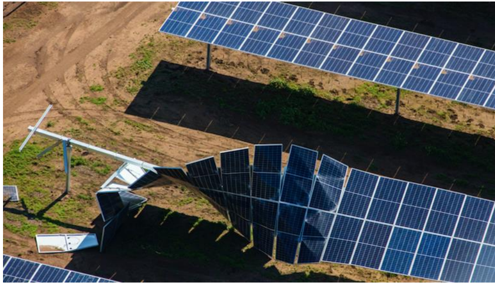
Figure 1.5. Solar tracker after failure. Oakey 2 Solar Farm. Oakey, Queensland, Australia (extracted from Gifford (2019))
