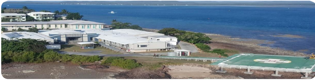
Figure 2.1 Thursday Island Hospital (Foster, 2017).
