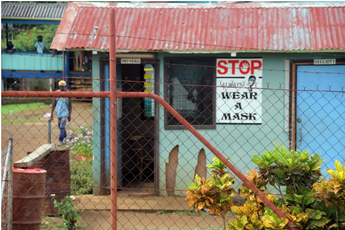
Figure 1.2.12 Daru General Hospital (photograph courtesy of Aaron Smith, 2015).
