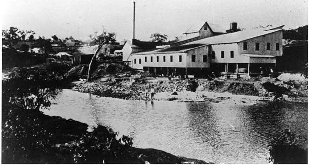
Plate 7. Great Northern Tin Mining Company's Battery, Herberton. [QGMJ, 14 May 1910]
