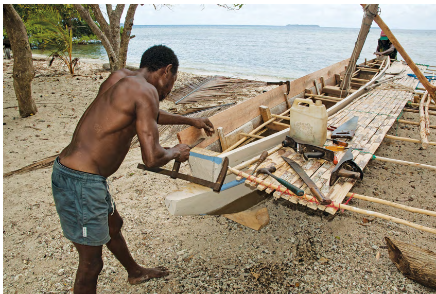
Figure 3.5: Sailau undergoing renovation on Tubetube Island, 2005
