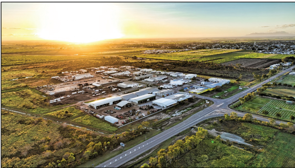
Figure 1. Aerial image of an area in Ayr, QLD by Burdekin Drones.
