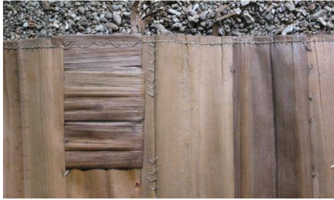
Plate 4.3.11: Mid-rib split repaired with bird's feet stitch, Yaga Settlement
