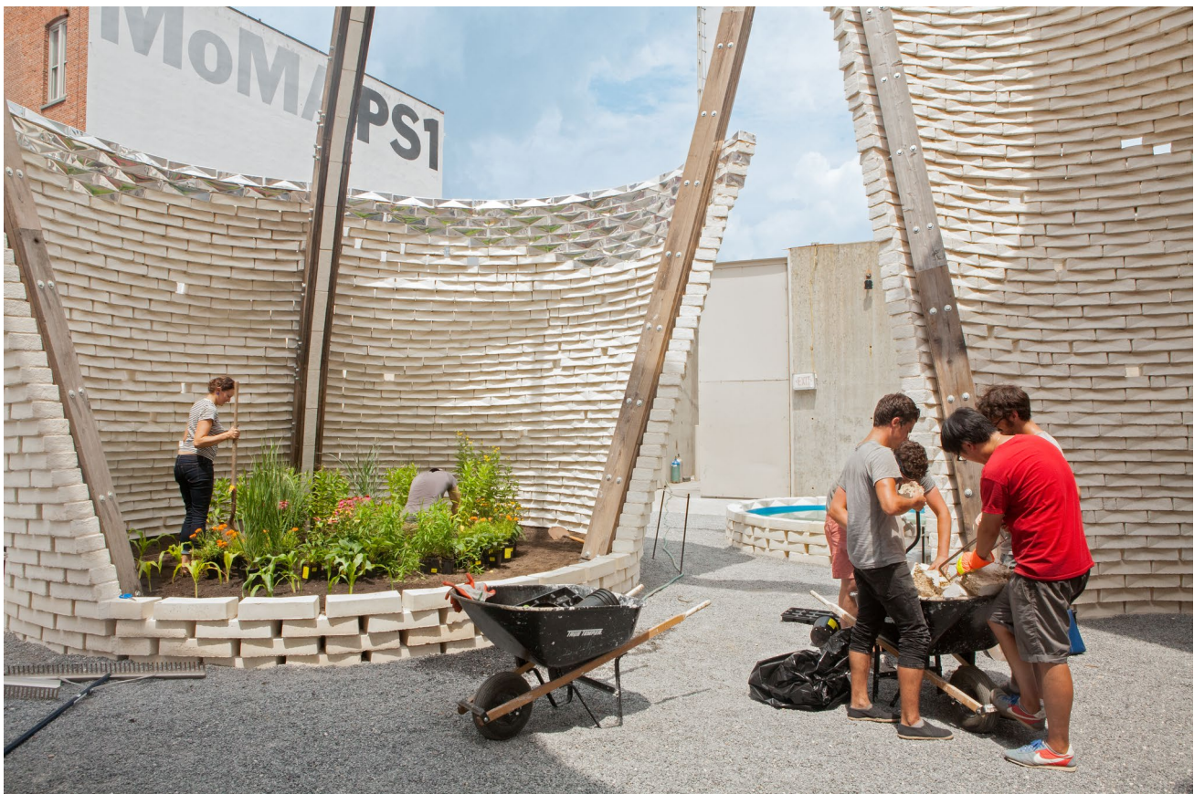
Fig. 1 Hy-Fi by The Living / David Benjamin, with structural engineering by ARUP. Commissioned by the Museum of Modern Art (MoMA) PS1, New York 2014. Photo courtesy of The Living
