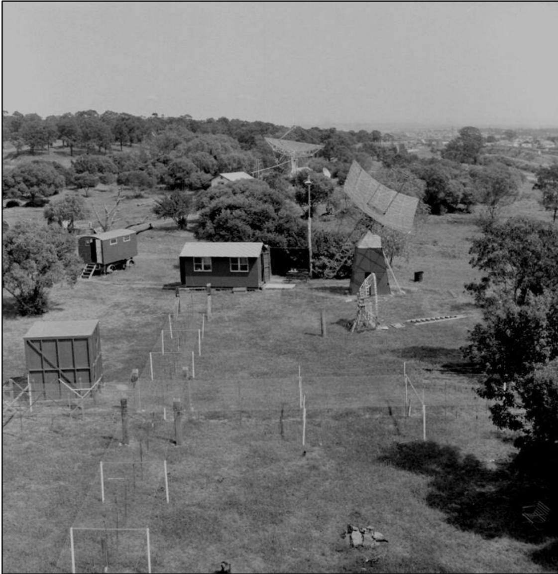
Figure 79: The Mills Cross Prototype at Potts Hill. In the background is the 16-ftx18-ft Paraboloid and the 36-ft Transit Parabola (Courtesy of ATNF Historical Photographic Archive: B3171-4 Image Date: 7 October 1953).
