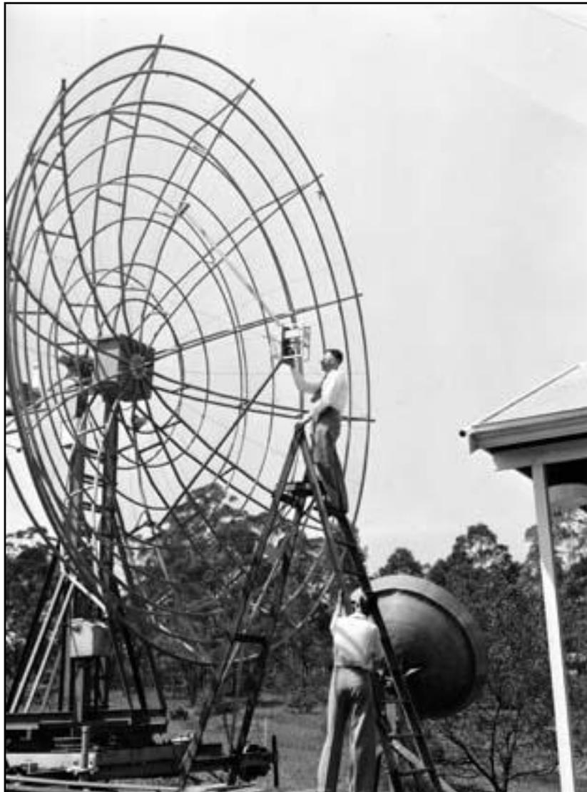
Figure 212: The 21-ft aerial at Murraybank with its new feed system. The smaller reference aerial is also visible in the background (Courtesy of the ATNF Historical Photographic Archive).
