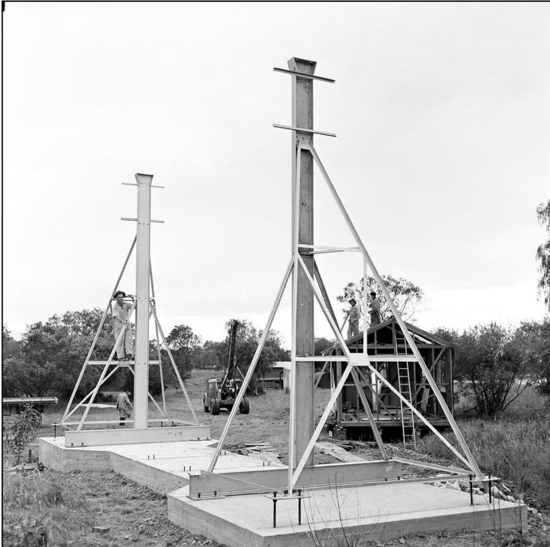
Figure 61: The two major support posts of the 36-ft aerial during construction (Courtesy of ATNF Historical Photographic Archive: B2778-5 Image Date: 19 June 1952).
