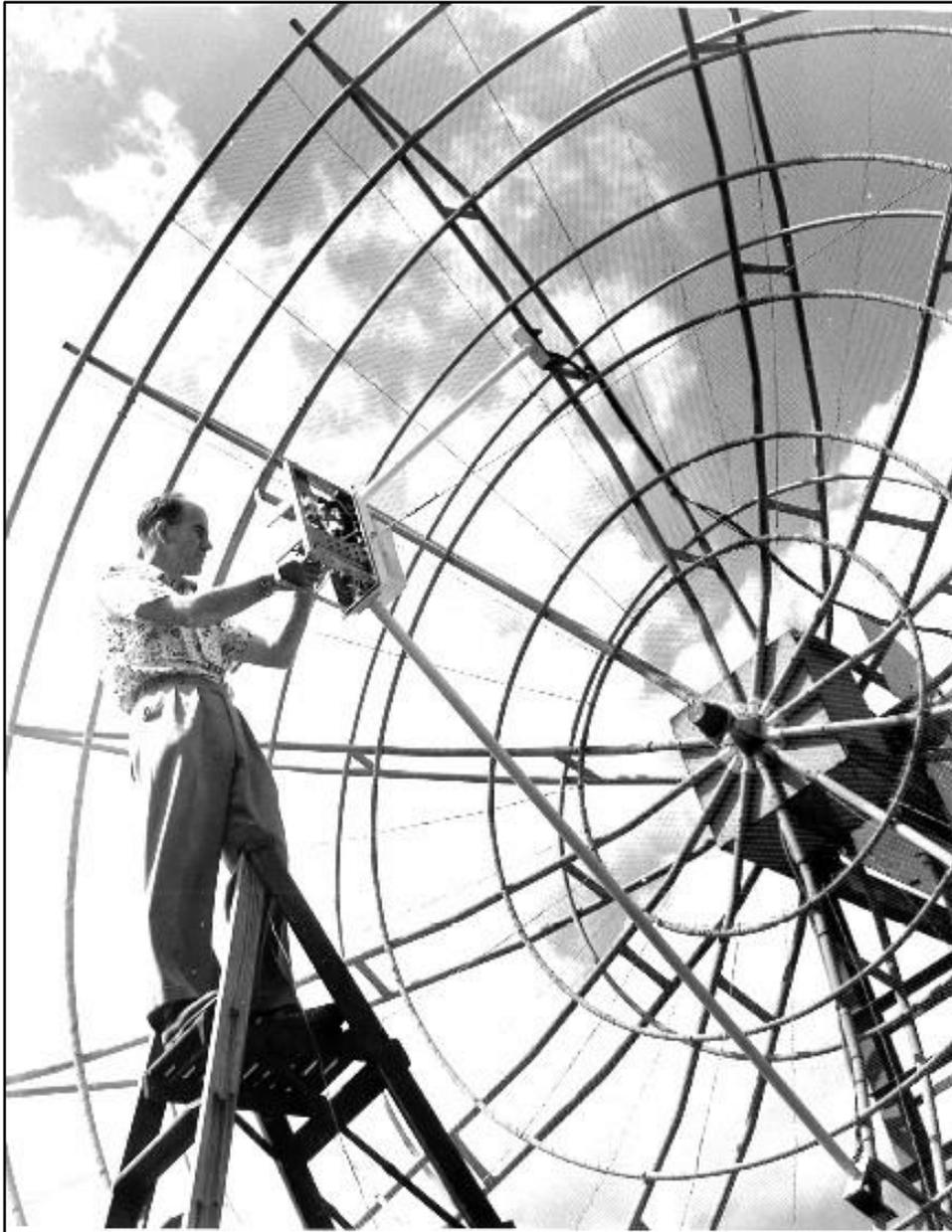
Figure 213: Dick McGee working on the primary feed of the 21-ft Murraybank aerial (Courtesy the ATNF Historical Photographic Archive: R5695-8).
