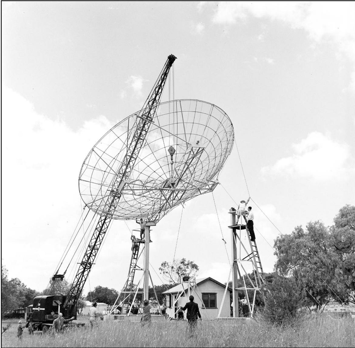
Figure 63: The 36-ft Parabola being lifted by crane into the transit mounting (Courtesy of ATNF Historical Photographic Archive: B2975-19 Image Date: 14 January 1953).
