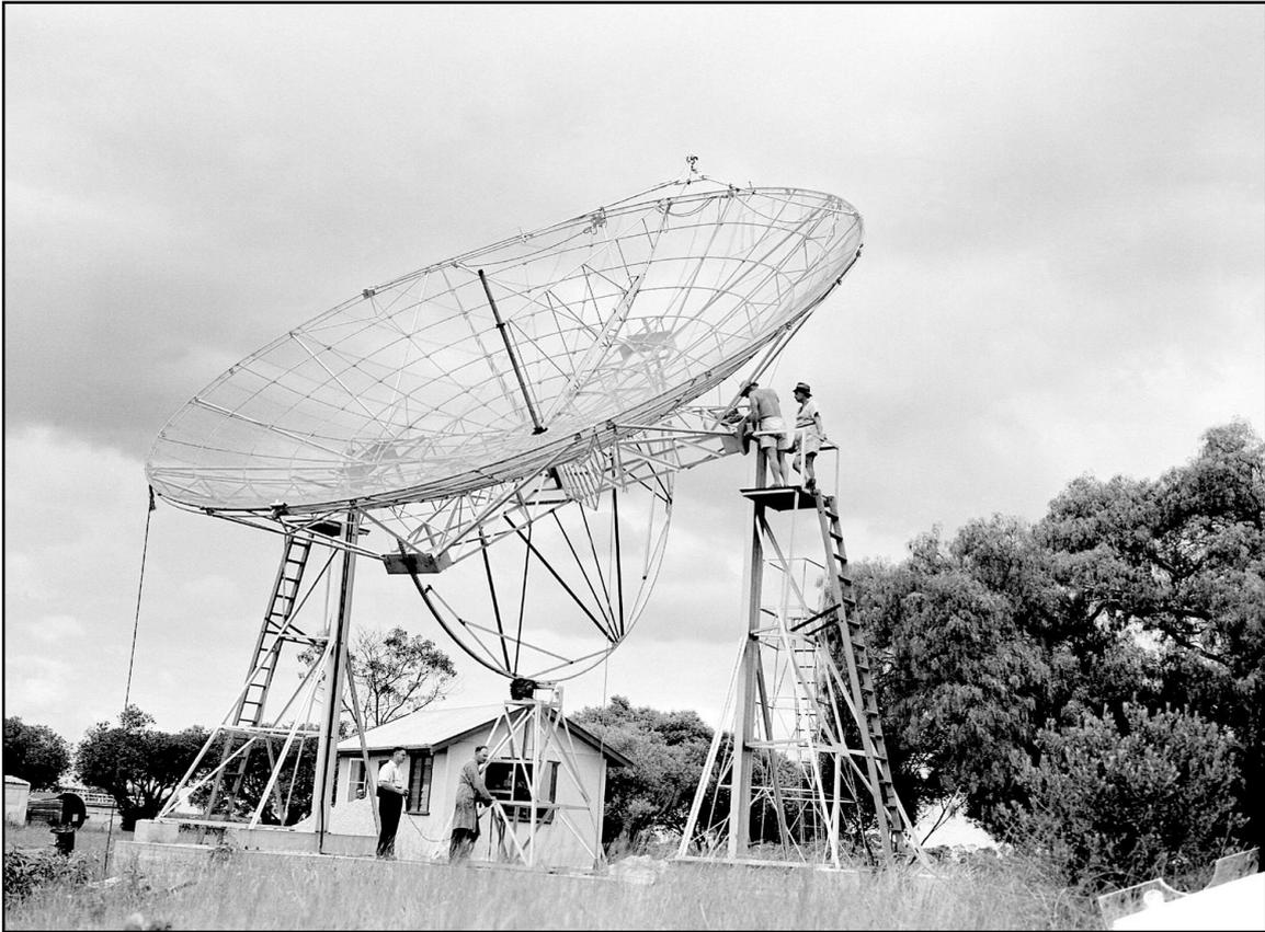
Figure 64: The 36-ft Transit Parabola in final assembly in its mounting (Courtesy of ATNF Historical Photographic Archive: 2975-21 Image Date: 14 January 1953).
