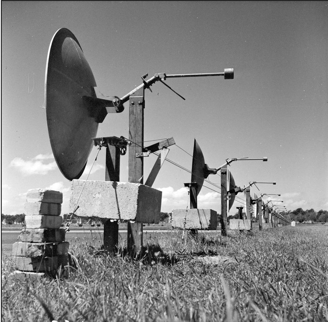
Figure 51: The array showing the bracing weights for the open-wire transmission lines (Courtesy of ATNF Historic Photographic Archive: B2976-1 Image Date: 28 November 1951).
