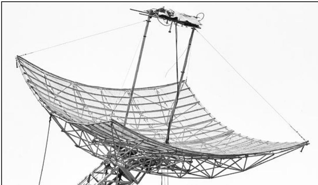
Figure 34: 16-ft  $\times$  18-ft Paraboloid showing guide wires supporting the prime focus receiver plate (Adapted from ATNF Historic Photographic Archive: B2649-3 Image Date: 2 January 1952).
