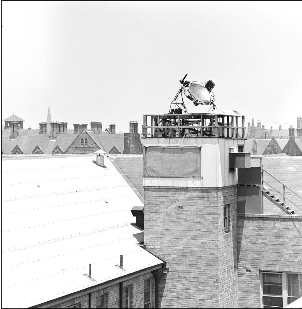
Figure 40: The ex-Searchlight 44" Paraboloid shown mounted on the 'Eagle's Nest' on top of the Radiophysics building in the grounds of Sydney University (Courtesy of ATNF Historic Photographic Archive: B1641 Image Date: 4 January 1949).
