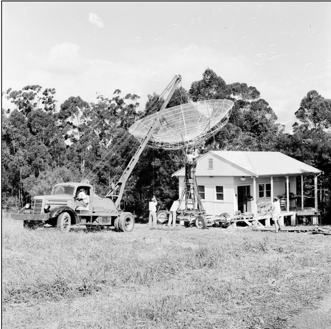
Figure 211: The 21-ft aerial being installed at Murraybank in 1956. The equipment hut is in the immediate background (Courtesy of the ATNF Historical Photographic Archive: B3973-4 Image Date: 18 May 1956).
