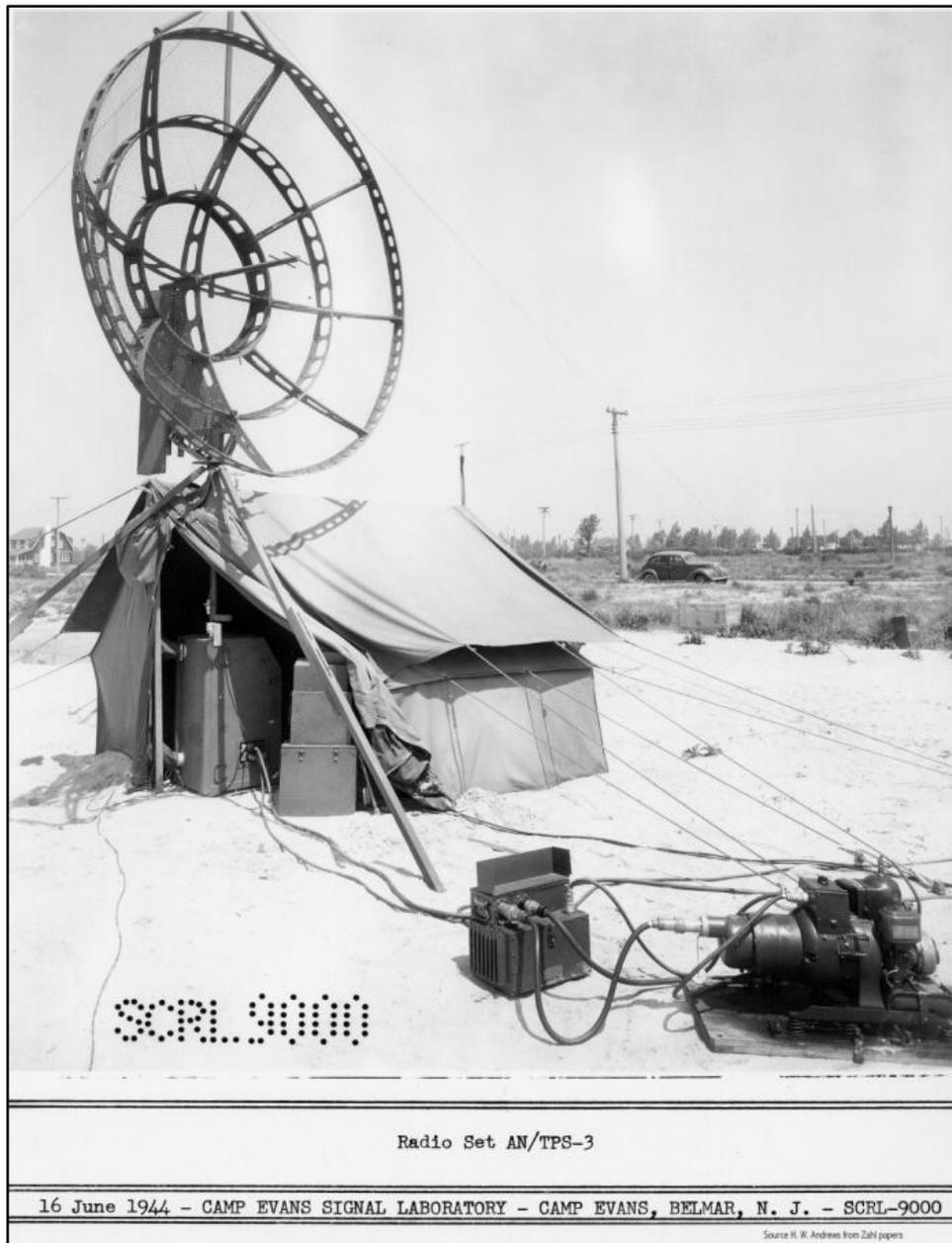
Figure 37: AN/TPS-3 Radar Set in operation on 16 June 1944 at the Camp Evans Signal Laboratory, U.S. Army Signal Corps. (Courtesy of CE LCMS Historical Office Department of the Army, USA.)
