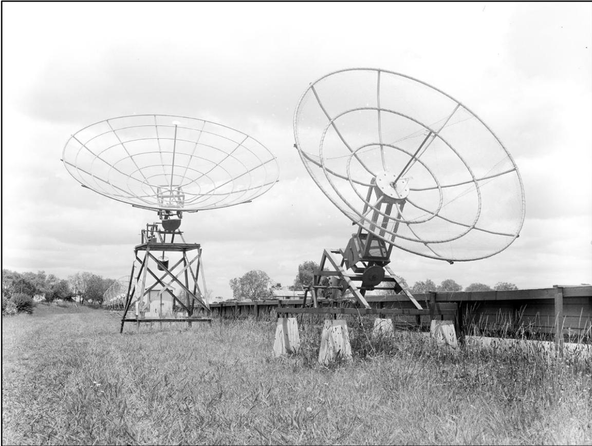
Figure 58: The prototype of the larger aerial in the background that was to be used in the new crossed array being tested at Potts Hill (Courtesy of ATNF Historical Photographic Archive: B3881-2 Image Date: 13 December 1955).
