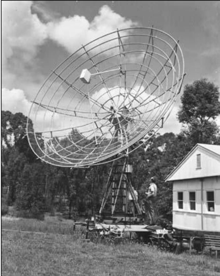
Figure 74: The 21-ft Parabola at the Murraybank field station (Courtesy of ATNF Historical Photographic Archive).
