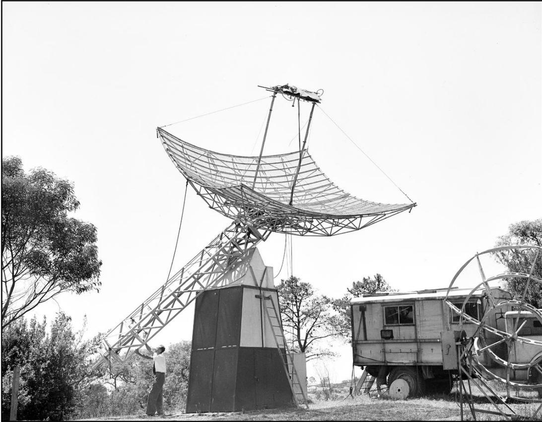
Figure 31:16-ftx18-ft Paraboloid on the new polar mount at Potts Hill field station (Courtesy of ATNF Historic Photographic Archive: B2649-3 Image Date: 2 January 1952).
