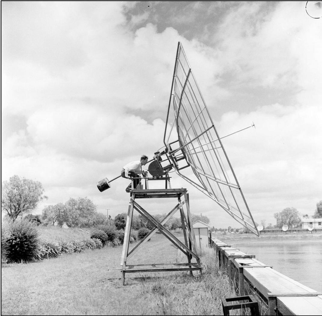
Figure 59: Another view of the cross grating prototype aerial being tested at Potts Hill (Courtesy of ATNF Historical Photographic Archive: B3881-14 Image Date: 13 December 1955).
