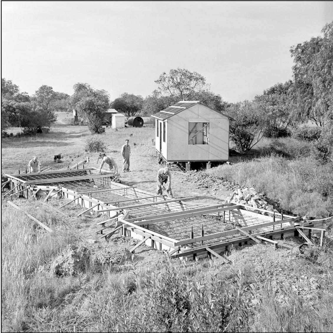
Figure 60: Construction of the foundations for the 36' Transit Parabola (Courtesy of ATNF Historical Photographic Archive: B2768-1 Image Date: 6 June 1952).
