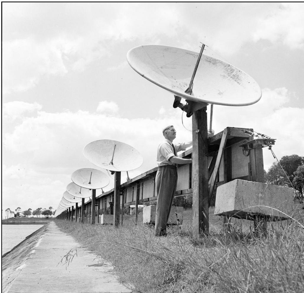
Figure 50: The 32-element array at Potts Hill (Courtesy of ATNF Historic Photographic Archive: 2976-1 Image Date: 14 January 1953)
