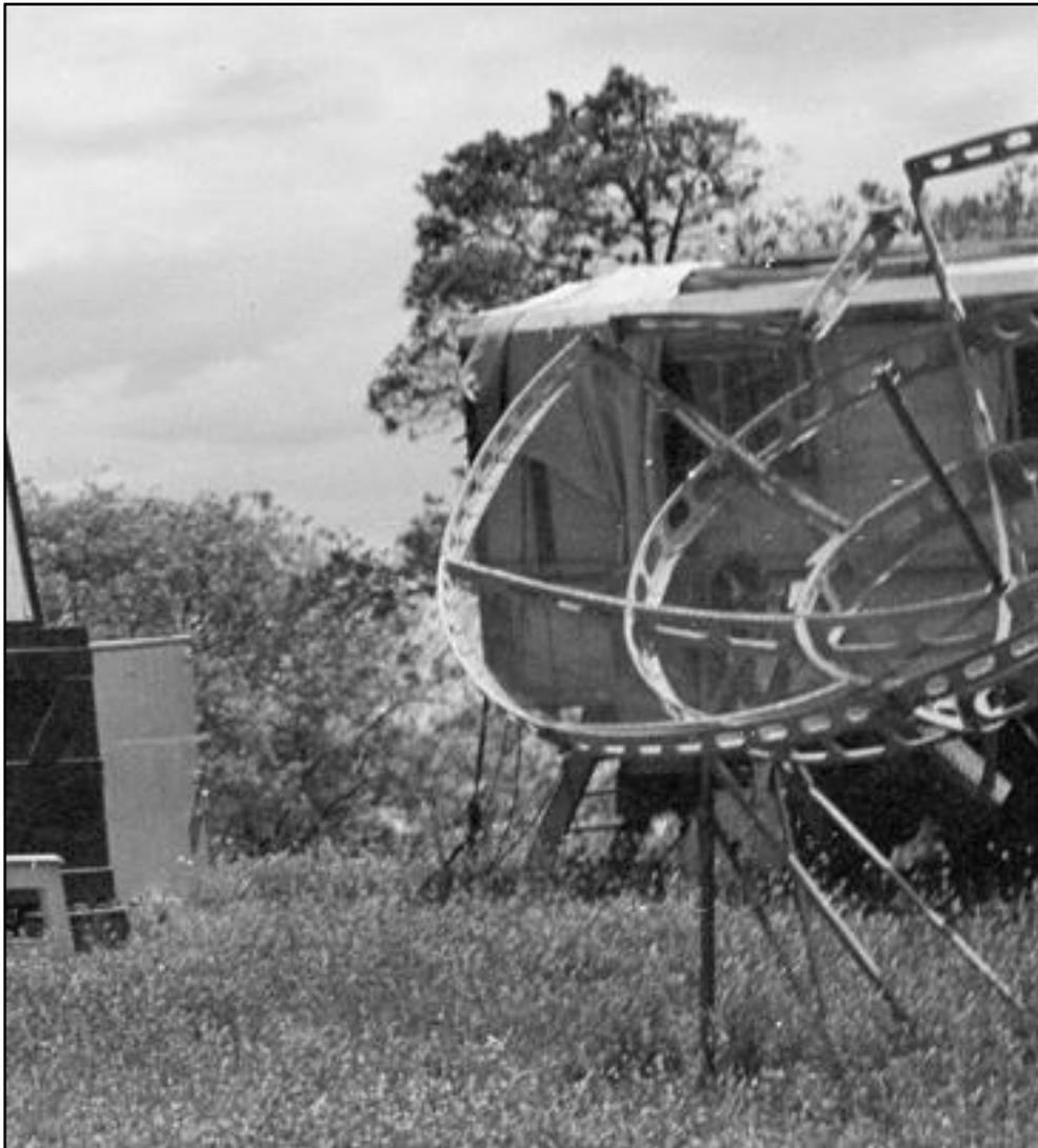
Figure 82: A 10-ft Parabola showing damage to one of its eight sections at Potts Hill in the 1950s (Adapted of the ATNF Historical Photographic Archive: B2639 Image Date: 28 November 1951).
