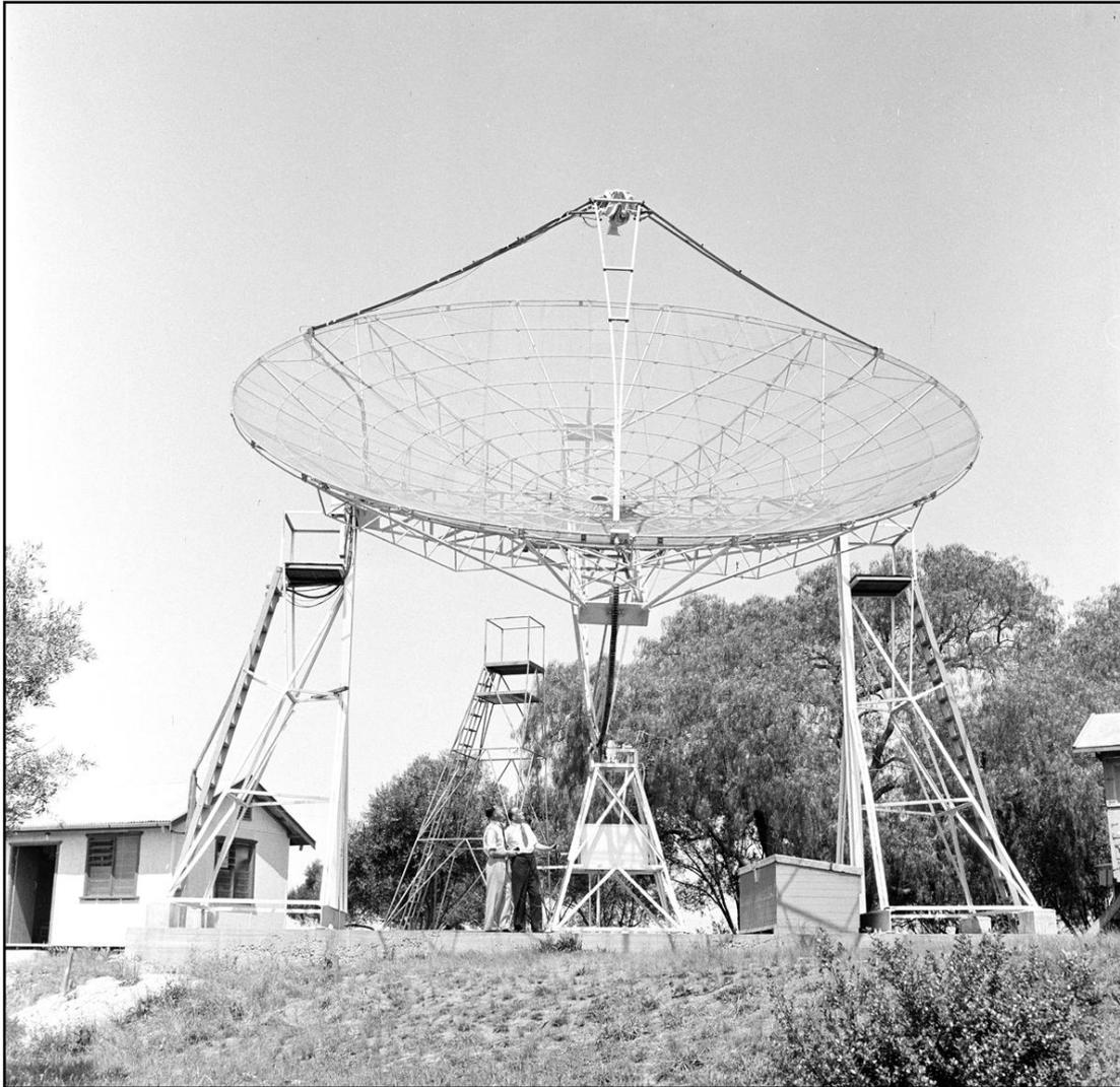
Figure 66: The 36-ft Transit Parabola ready for H-line observations (Courtesy of ATNF Historical Photographic Archive: 3170-2 Image Date: 14 January 1953).
