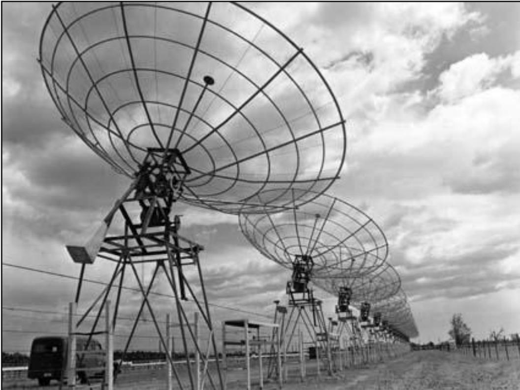
Figure 208: The Chris Cross at Fleurs Field station. The Murraybank aerial was based on this aerial design with an increased diameter and strengthened structure (Courtesy of the ATNF Historical Photographic Archive).
