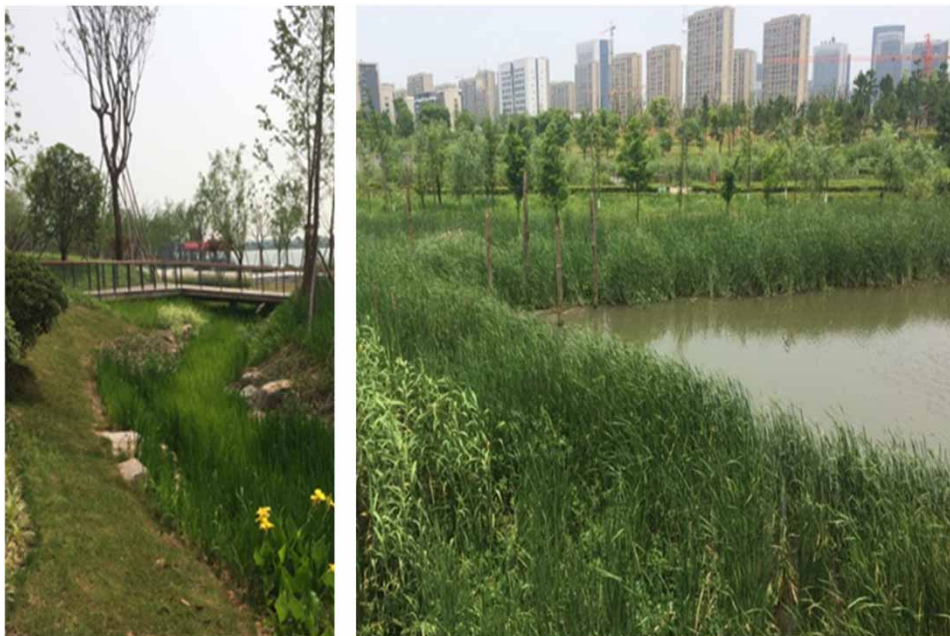
Figure 2 | SCP infrastructure in Jiangbei District, Ningbo. Bio-swale (left) and artificial wetland (right) (Source: Authors).
