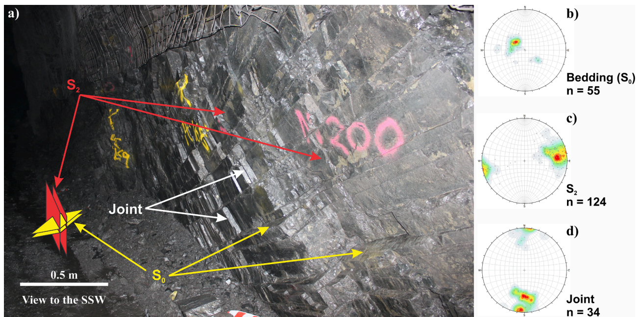
Fig. 5. A) Large amplitude F_1 and F_2 Type 1 interference fold preserved in a low strain domain in the North Mine (grid reference 3B). Here, over successive levels, the interaction of three prominent planes results in the development of rhomboid blocks. Photo was taken in the approximate position of the main shear zone. b, c, d) Equal angle, lower hemisphere stereoplots of S_0 (b), S_2 (c) and joint (d) from levels N125 – N220 (125 – 220 m below surface). S_0 has a consistent southeast dip and small-scale low-angle thrusts are developed within the beds and propagate between them. Steep, S_2 undulates with dominant west dips and is marked by thin, sulphide veins, which combined with the chlorite alteration, causes slabbing along the S_2 planes. The joint set has a general north dip and occurs orthogonal to the bedding.
