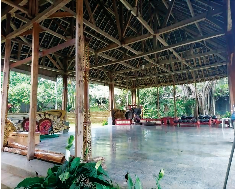
Figure 1. Main Pavilion of the Mangun Dharma Art Studio; (source: Doc. Dani, 2018).
