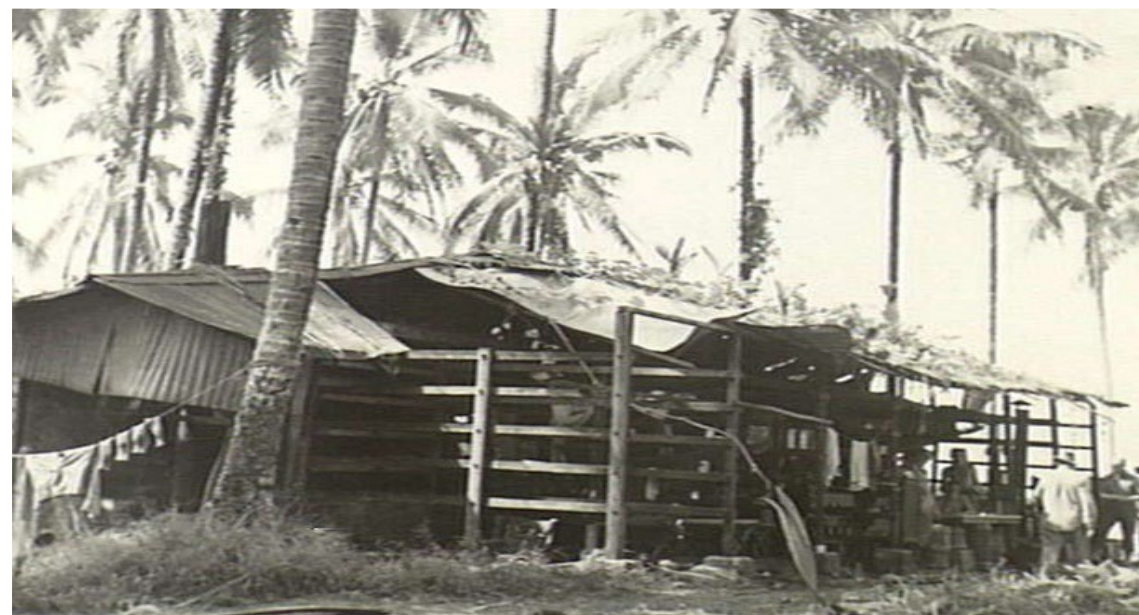
Figure 11. An old copra drying shed on Palmalmal Plantation which had been used as a Japanese kitchen during the occupation, 21st November 1944. Image credit: Australian War Memorial 077159 https://www.awm.gov.au/collection/C20333
