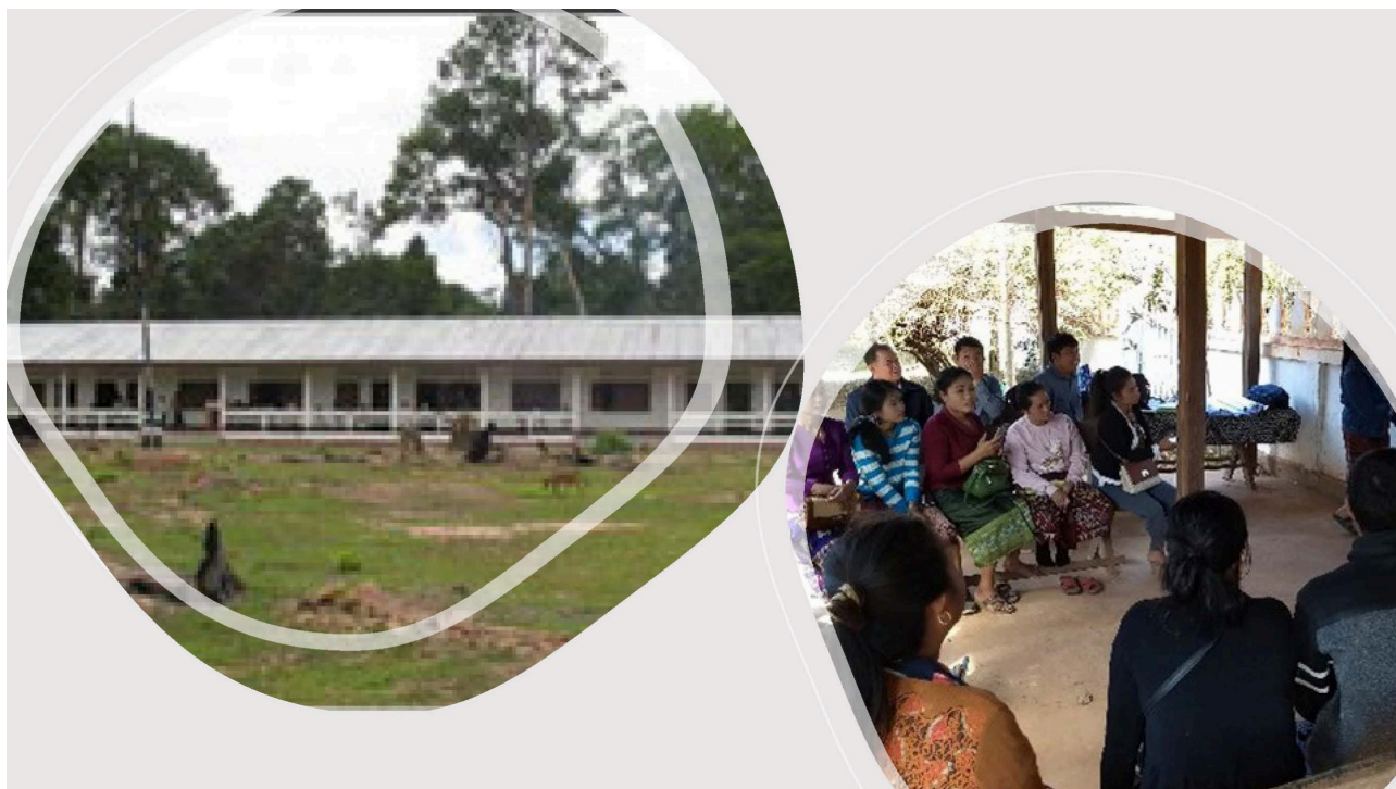
Figure 21. The District Development Fund (DDF) instituted by UNDP enabled planning at local level to identify projects, including at village and later District level. Most projects were concrete infrastructure such as schools (as in the example depicted here). This image by John Connell is licensed under CC BY (Attribution) 4.0
