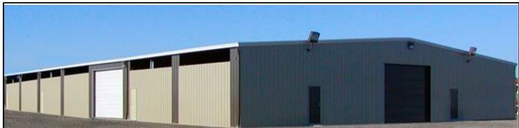
Figure 1.1: Typical large span industrial type building
