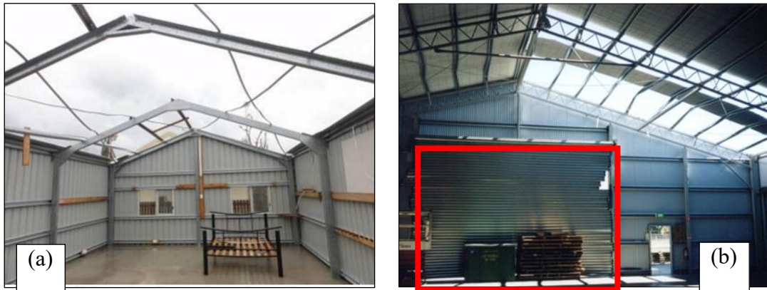
Figure 1.3: Structural damage to industrial buildings (a) Loss of entire roof - CTS Report TR57 (b) Windward roller door failure –Stehle and Henderson (2001)
