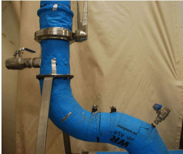
Figure 4.5; Pipe before sample container, including instrumentation ports and bypass valve.
