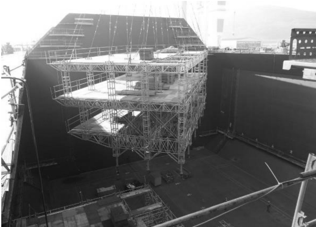
Figure 13. Cargo Hull Scaffolding Being Lowered into Place in One of the Ship's Four Cargo Hulls, South Korea.
