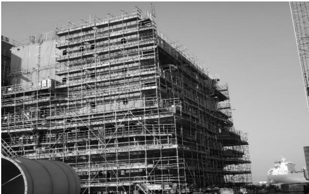
Figure 16. Accommodation Block for a Ship is Under Construction With Over One Million Scaffolding Pieces Required for Construction, South Korea.
