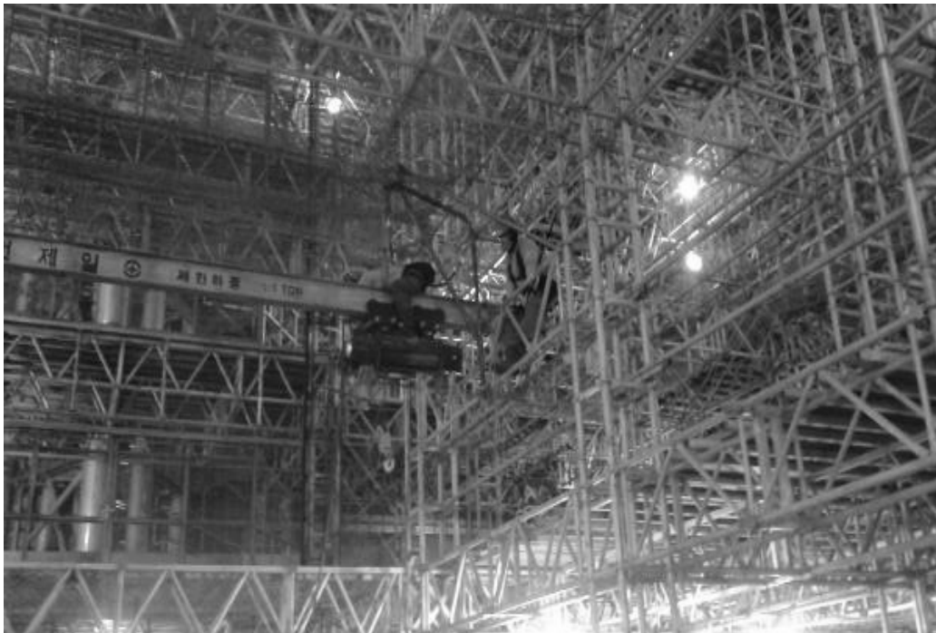
Figure 14. Cargo Hull Scaffolding Being Dismantled by Workers 40 Metres Above the Ship's Deck Floor, South Korea.
