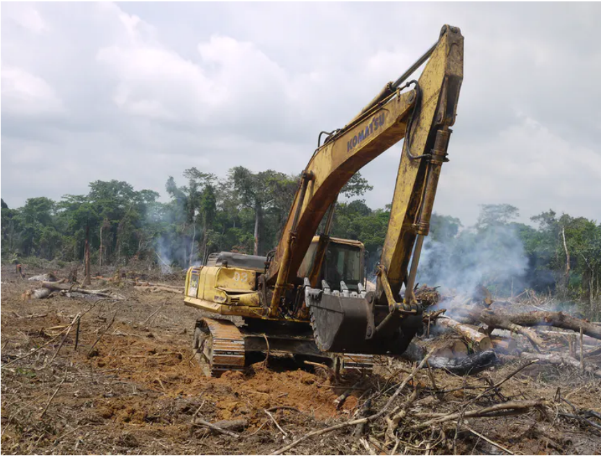
China-funded road-construction project in the Congo Basin. William Laurance
