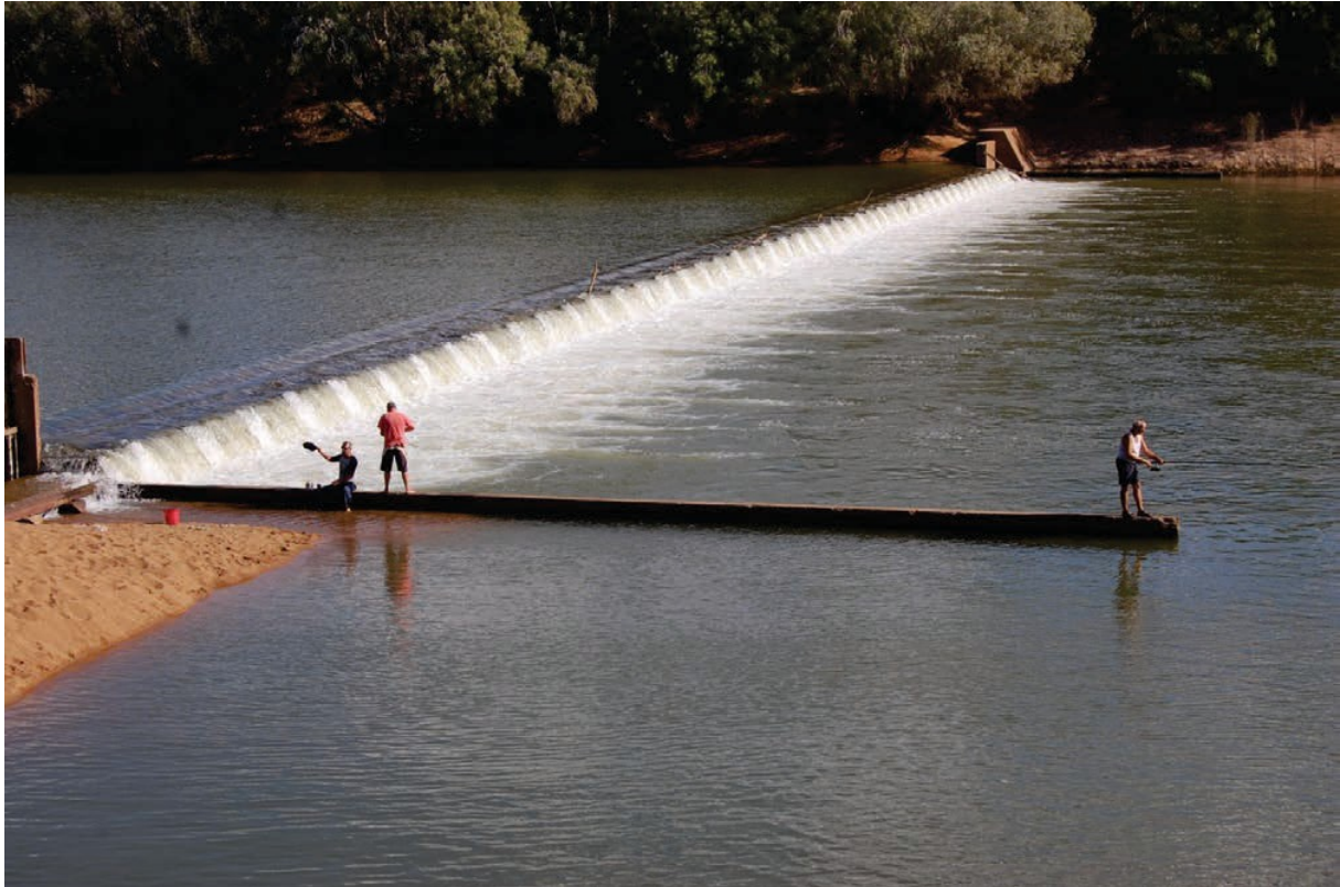
The Fitzroy River barrage, Camballin irrigation scheme. © David Morgan
