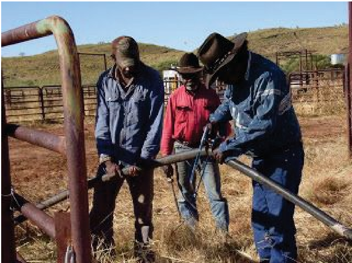
Station workers cutting and joining the poly pipes for the trough in the yard; Eugene, Steven, and Roy at Beaton's bore yard at Millijiddee Station. © Benjamin Laurel, Wulungarra Community School blog
