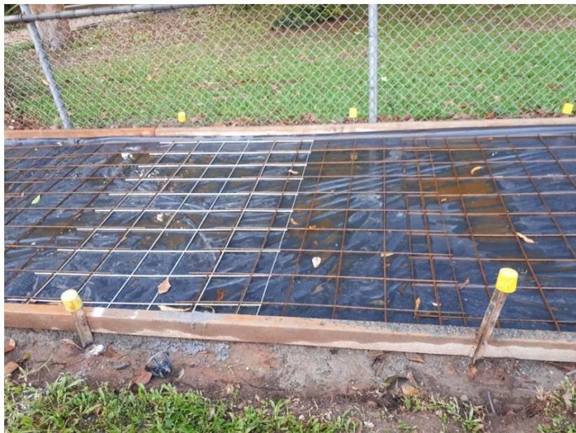
**Figure 7.2 Reinforcing mesh for concrete footpath**
