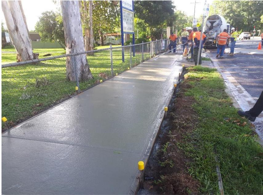
**Figure 7.8 Curing of freshly placed concrete**
