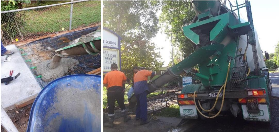
**Figure 7.4 Ready mix concrete pouring**
