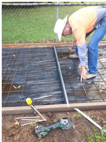
**Figure 7.3 Form work and reinforcement arrangement prior to concrete pour**
