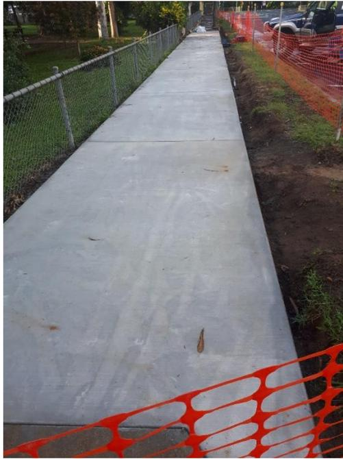
**Figure 7.10 RGS 40 – TMR concrete footpath**
