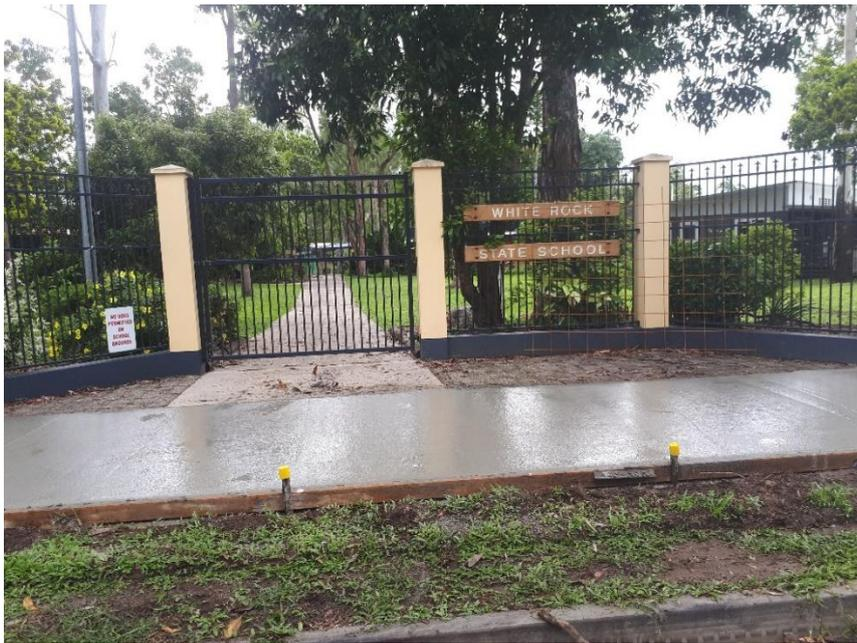
**Figure 7.9 Footpath in the fresh stage**
