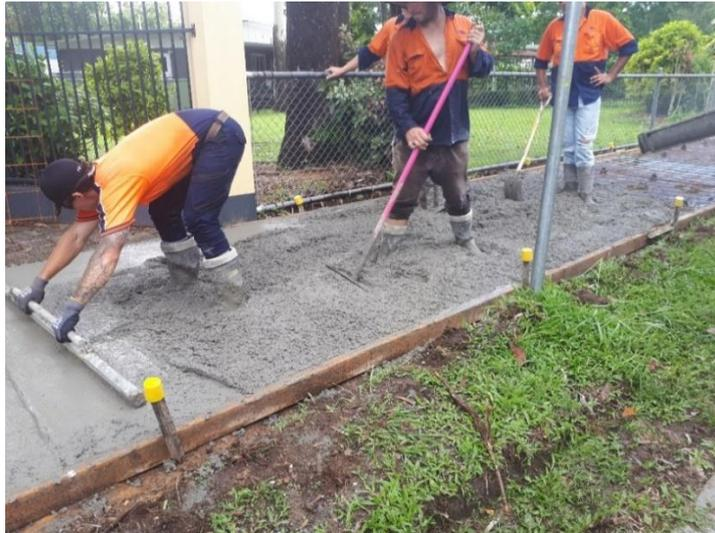
**Figure 7.6 Screeding of the concrete mix**
