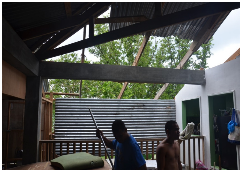
Plate 6.3 Remains of the roof structure, 6 November, 2013. (D.Tibbetts)
