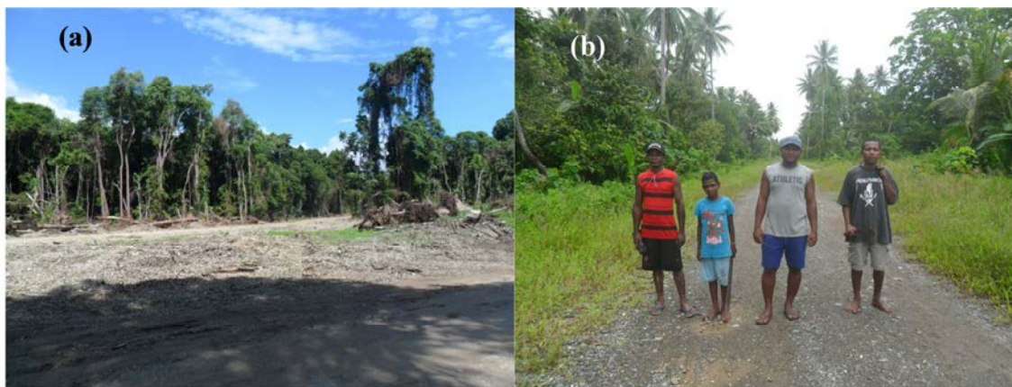
Figure 4.19: (a) A road under construction in the study area. (b) A previous coconut plantation that has been converted into road
