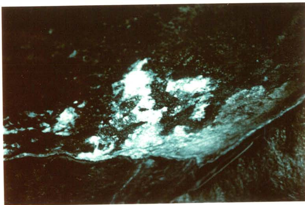
PLATE 4 Probable calcium oxylate deposit, exhibiting typical black layer in association with white crystalline deposit.
