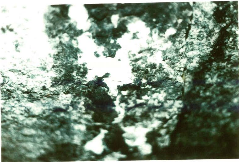
PLATE 3 Detail of damage associated with salt efflorescence. This type of photograph is useful for monitoring the deterioration of painted and engraved images.
