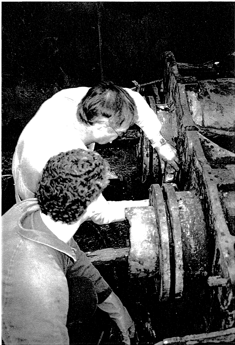
Figure 112a: The separation of the cylinders began with the insertion of a hydraulic jack.
