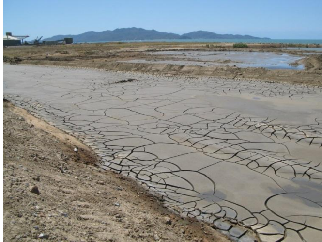
Figure 5.10 - Desiccation shrinkage cracks of dredged material in containment pond – eastern reclamation area- The Port of Townsville
