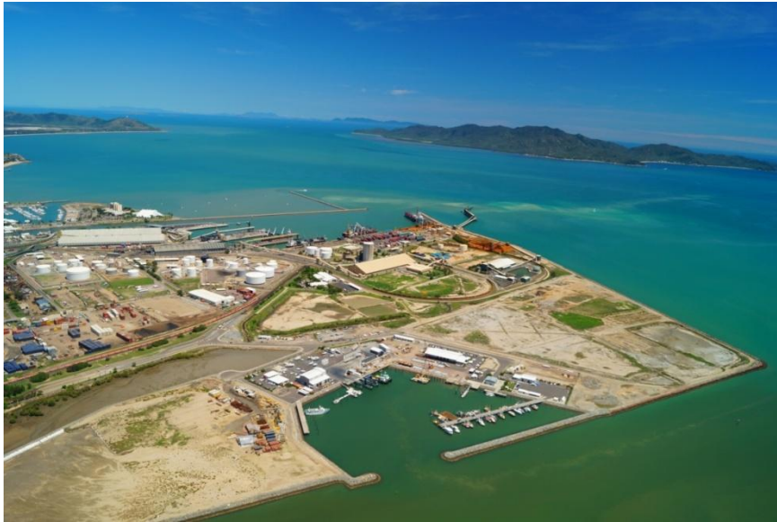
Figure 7.1 - Aerial view of the Port of Townsville's eastern reclamation area
