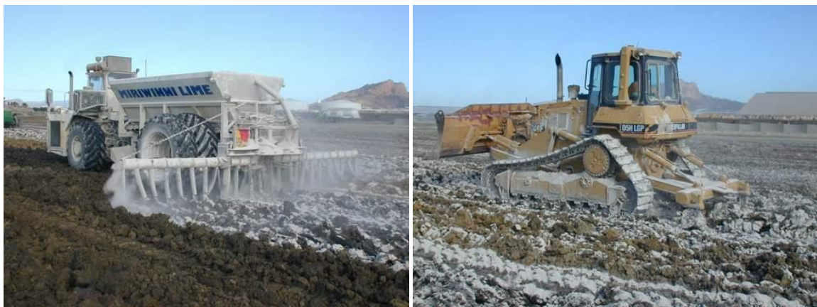
Figure 2.9 – Dredged material stabilisation with lime at the eastern reclamation area – the Port of Townsville (2007) (image courtesy of the Port of Townsville)
