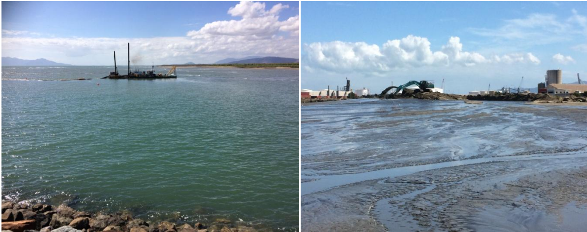
Figure 1.1- Dredging and dredged material placement operation at Port of Townsville – June 2017
