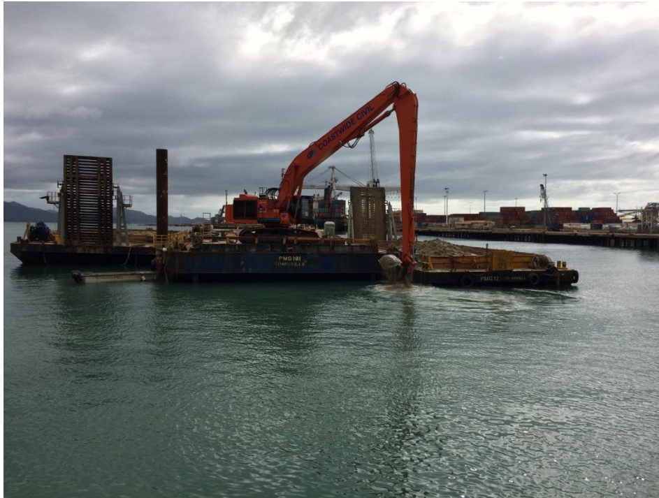
Figure 2.6 – Backhoe dredge deepening berth 7 pocket – the Port of Townsville (2015)
