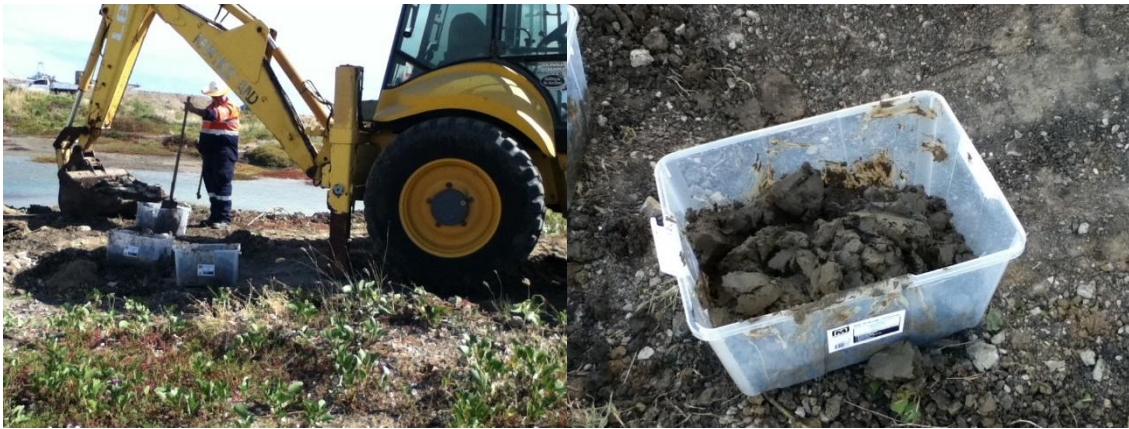
Figure 3.1 – Dredged material excavation– eastern reclamation area -the Port of Townsville
