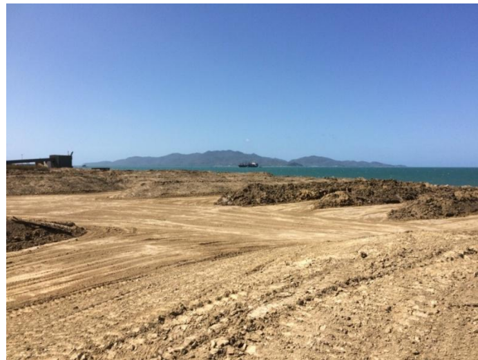
Figure 2.10 – Surcharging of eastern reclamation area – the Port of Townsville (2017)
