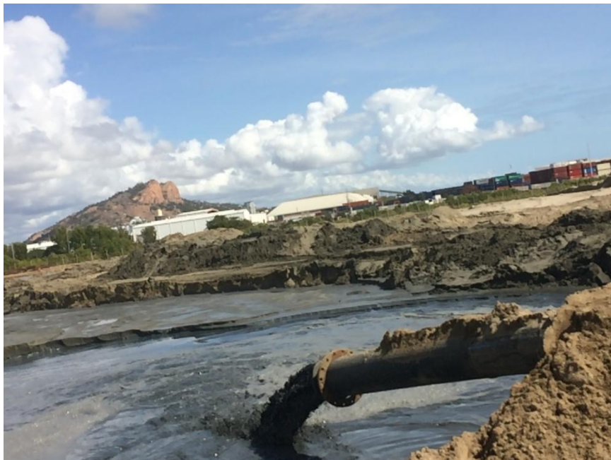
Figure 2.7 – Maintenance dredged material placement into land reclamation containment pond – eastern reclamation area the Port of Townsville (2017)
