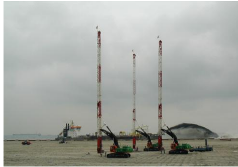
Figure 2.11 – Reclaimed land stabilisation with Prefabricated Vertical Drains – Chek Lap Kok airport land reclamation, Hong Kong (Kolman 2012)
