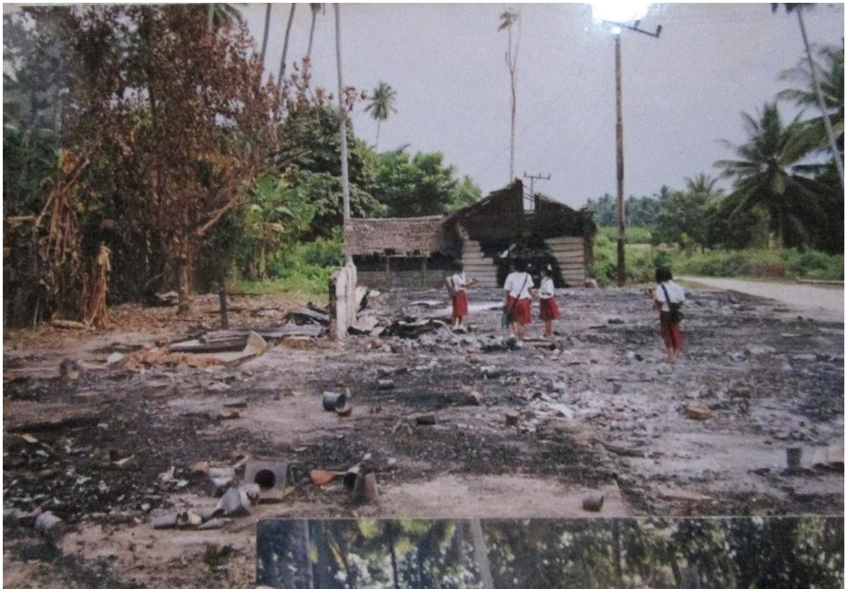
Figure 7: A school that was burned down in Aceh, Indonesia
