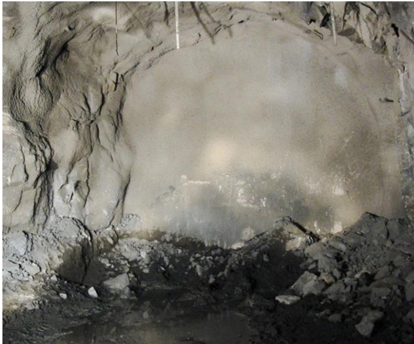
Fig. 2.4 Shotcreted barricades for a paste fill stope
