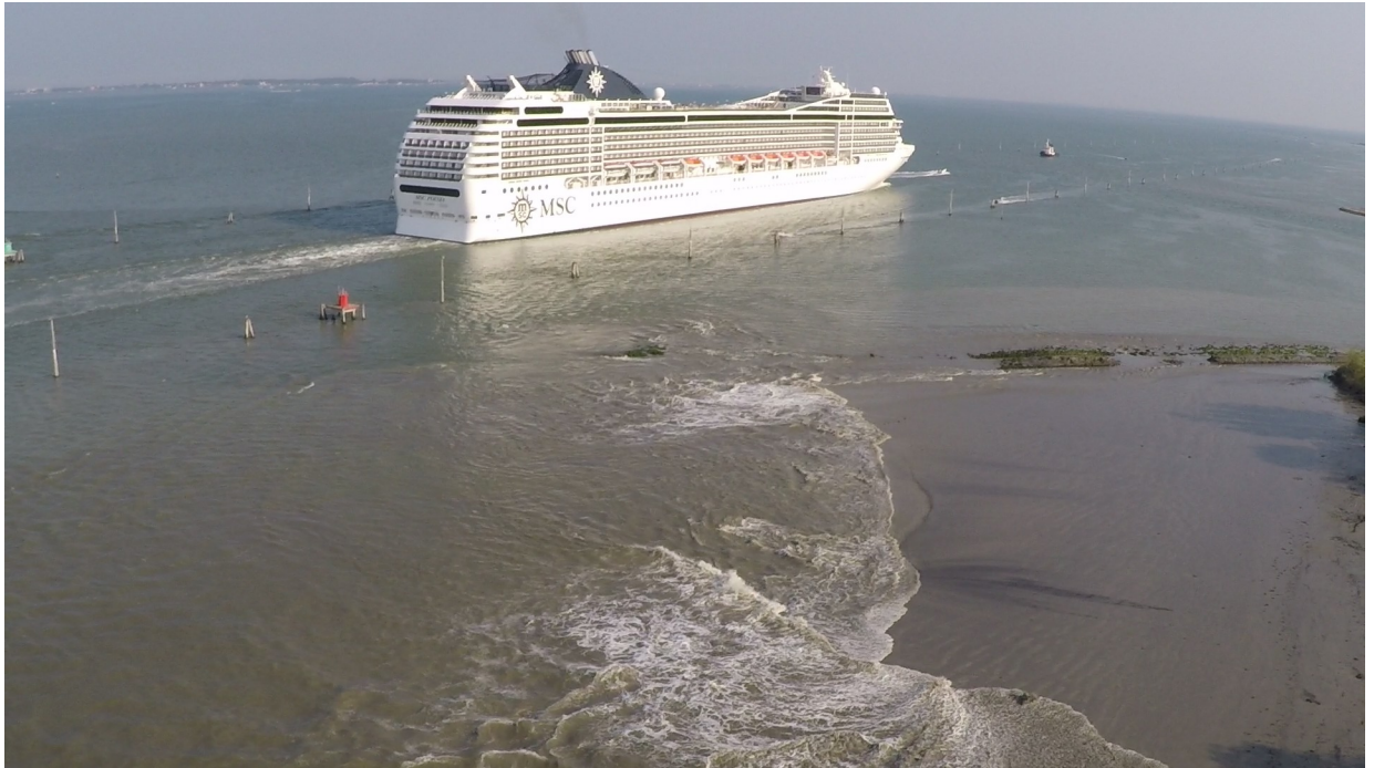
Fig 5. Aerial view of a cruise ship transit in the MMC. The depression wake exposes the collapsed materials of the original rip-rap revetment of the embankment at the southern end of the Cassa di Colmata B (CC-B). Image source: author's picture.
