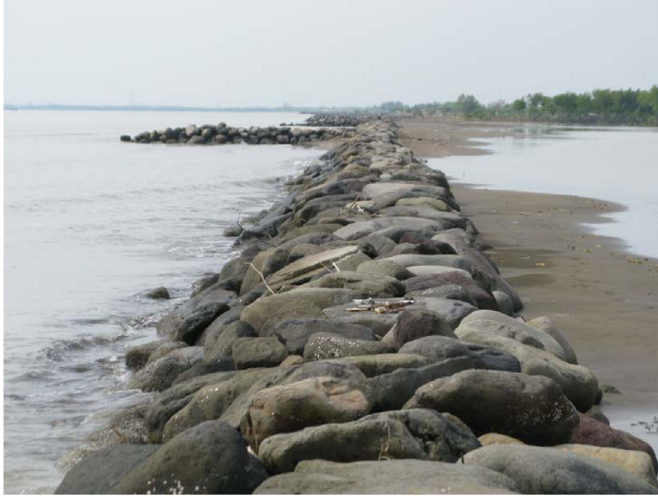
Figure 12: Rock wall was constructed to dissipate the energy of strong waves in Randusanga kulon
