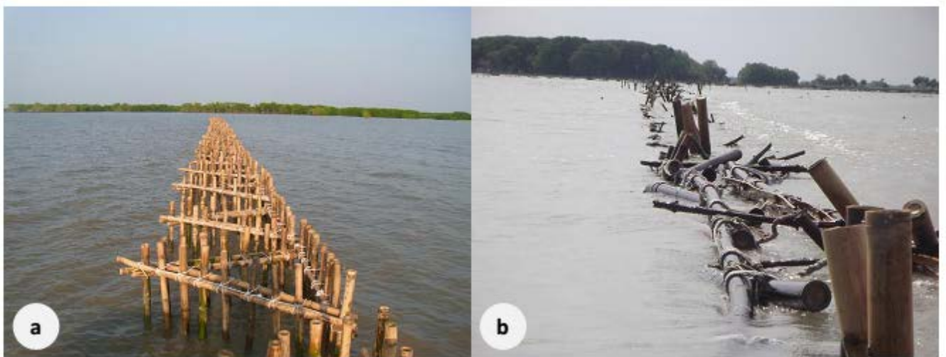
Fig 29: Triangular bamboo fences were constructed offshore in Sawojajar to protect seedlings from strong waves, a) new fences constructed 2011, and b) the fences were broken after construction in the same year.
