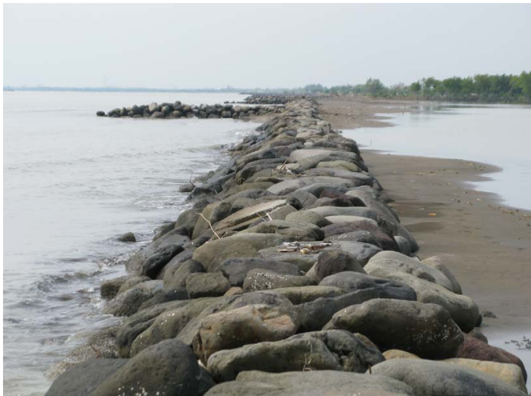
Fig 31: A rock wall was constructed to dissipate the energy of strong waves in Randusanga kulon.
