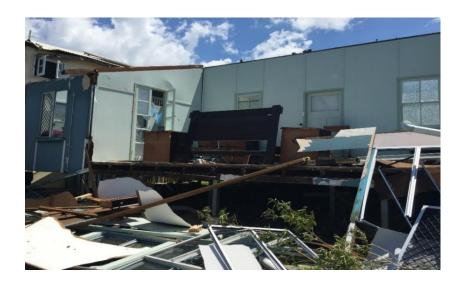
Figure 1.1. Roof removed and exterior walls collapsed in a pre1980's house at Yeppoon (photo courtesy of CTS)
