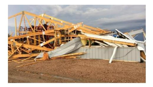
Figure 1.2. A metal-clad building with wood post frame construction destroyed (Prevatt et al., 2015)
