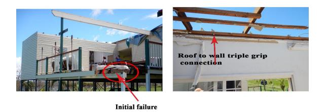
Figure 2.6. Roof loss after failure of windward side timber post (located at veranda) connection at floor (Photo courtesy of CTS)
