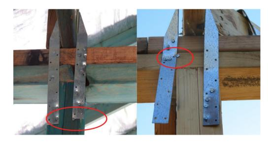
Figure 3.8. Common construction defects on the roof to wall strap connection
