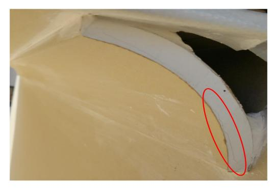
Figure 5.46. Hair-line crack on loading side ceiling cornice
