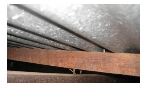
Figure 2.3. Partial withdrawal of nails in batten to rafter connection (Boughton et al., 2011)
