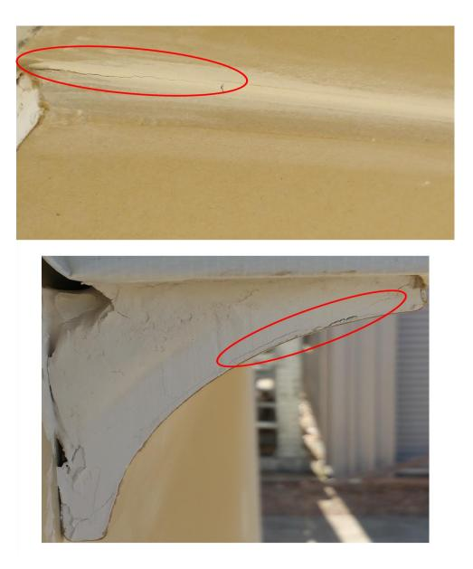
Figure 5.47. Hair-line crack on non-loading side ceiling cornice
