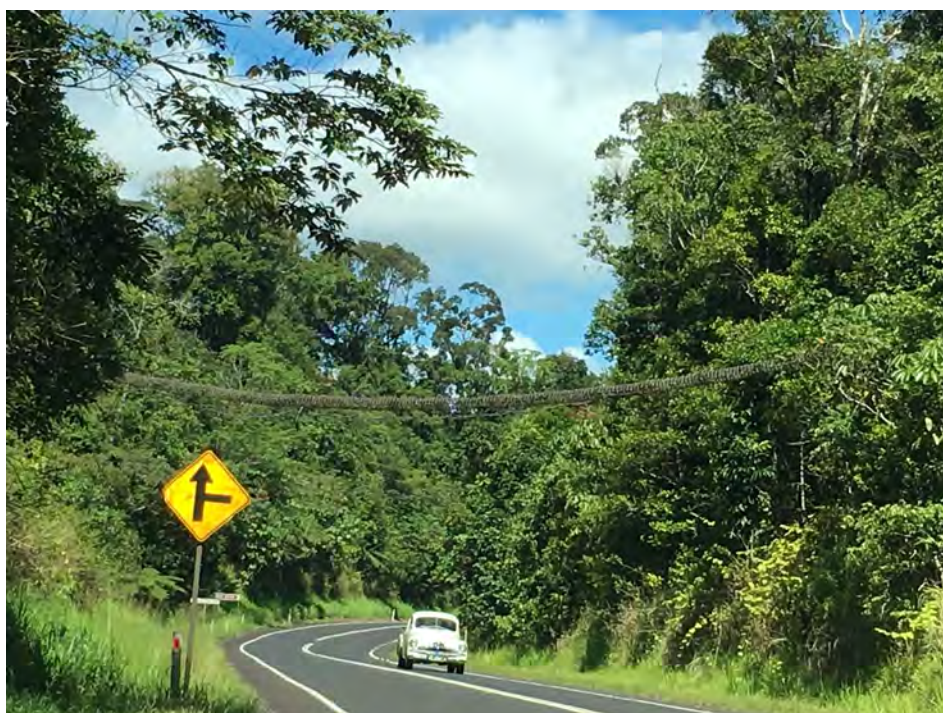
Mitigation measures such as these rope bridges across the Palmerston Highway in tropical far north Queensland, can assist in ameliorating the impacts of tropical roads on arboreal fauna species.
