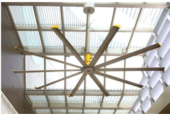
Fig. 2. Activated by human traffic, temperature and humidity, Smart fans will improve thermal comfort levels for residents. (Source: Housing and Development Board, 2014).
