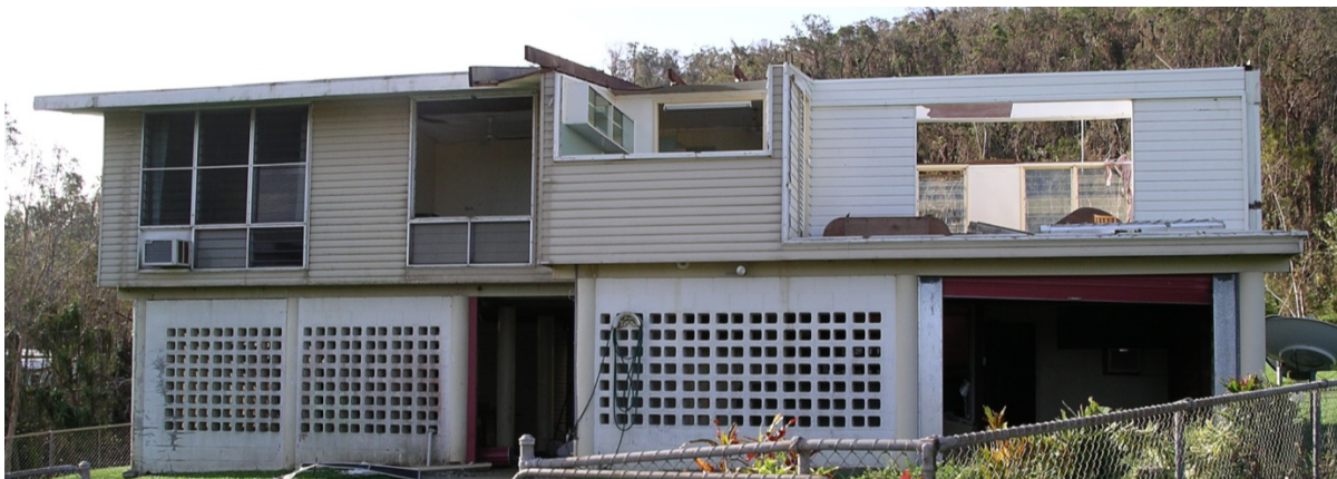
Figure 16. Roofing and wall damage to a high-set 1970s home as presented to builders, assessors, and engineers for experience based estimates of repair cost
