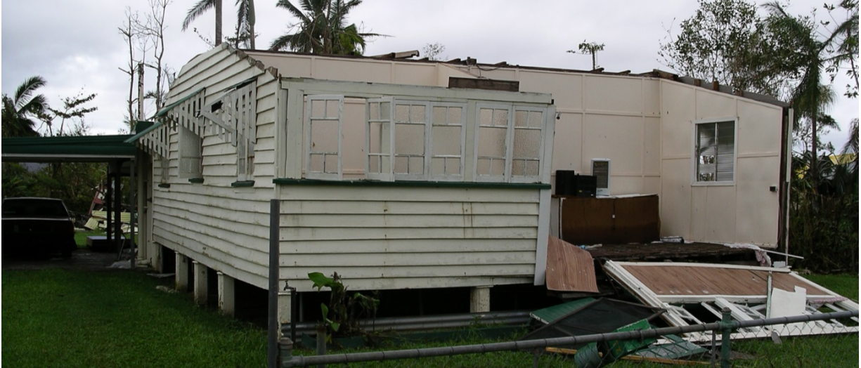
Figure 15. Roofing and wall damage to a low-set 1930s home as presented to builders, assessors, and engineers for experience based estimates of repair cost (high-set costs were also evaluated)
