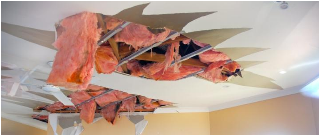
Figure 11. Wind driven rain damage to a modern (2000s) masonry block home as presented to builders, assessors, and engineers for experience based estimates of repair cost
