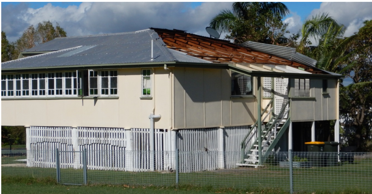
Figure 10. Wind-induced roofing damage to high-set 1920s home as presented to builders, assessors, and engineers for experience based estimates of repair cost
