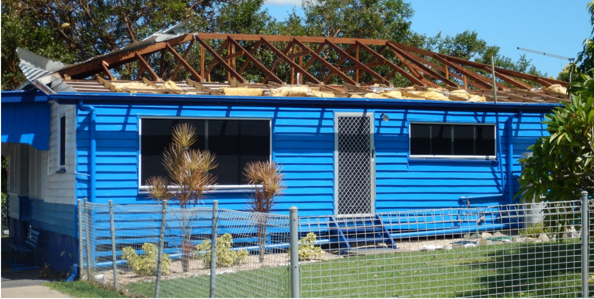
Figure 12. Wind-induced roofing damage to a low-set 1930s home as presented to builders, assessors, and engineers for experience based estimates of repair cost
