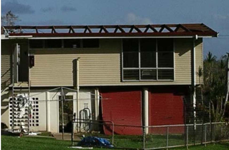
Figure 13. Wind-induced roofing damage to a high-set 1970s home as presented to builders, assessors, and engineers for experience based estimates of repair cost
