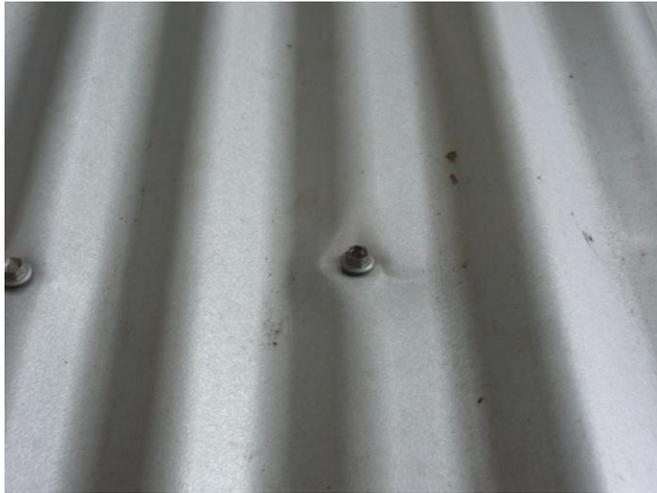
Figure 5.18: Plastic deformation of cladding around fasteners
