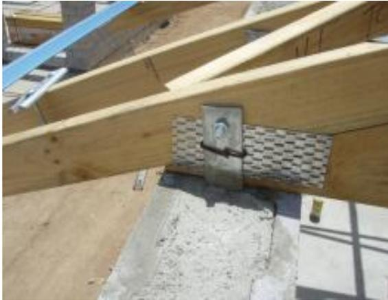
Figure 3.3: Truss-to-wall connection
