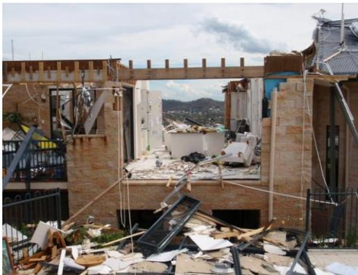
Figure 1.1: Damaged house from Brisbane thunderstorm (Leitch *et al.* (2010))
