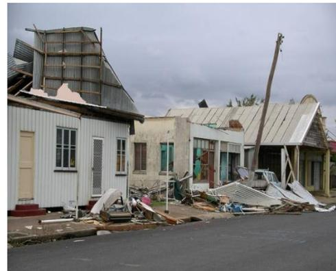
Figure 1.2: Building damage in Cyclone Larry (Henderson *et al.* (2006))
