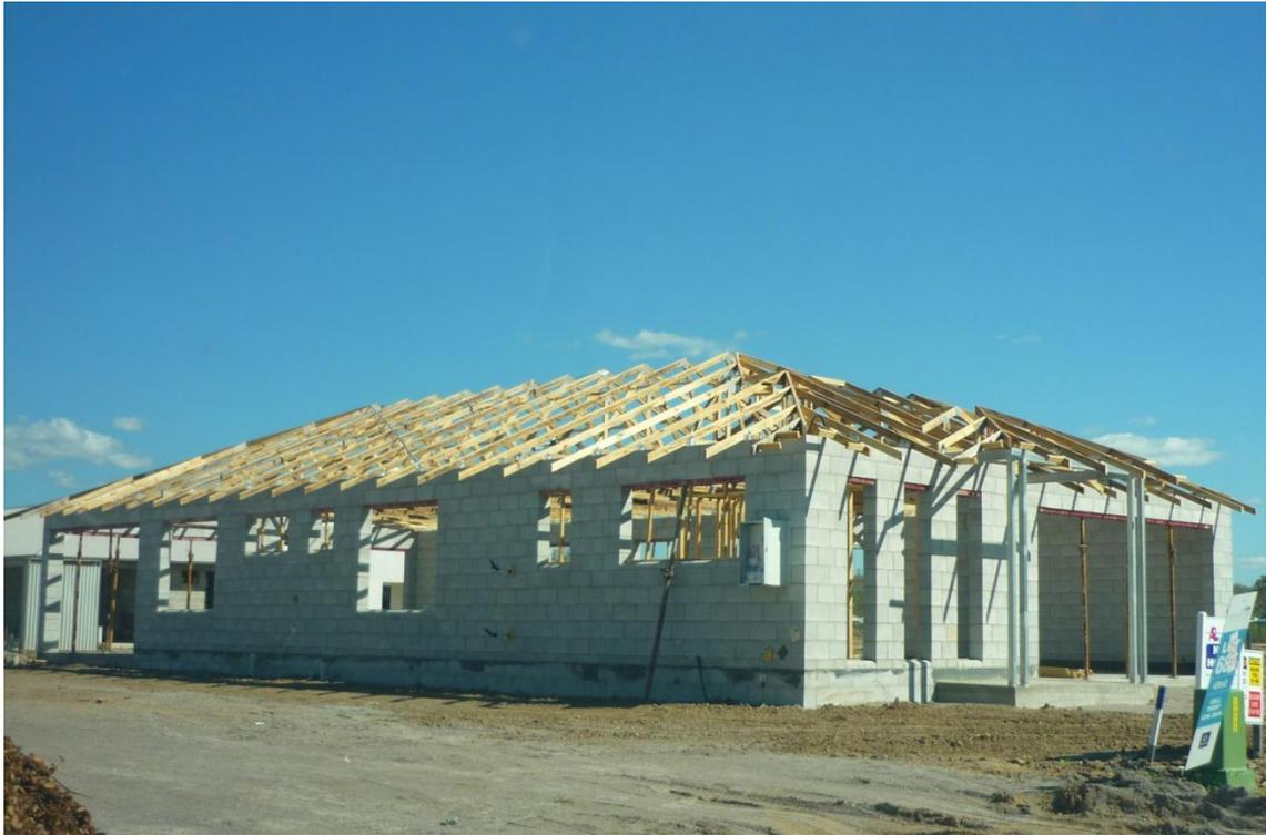
Figure 3.1: Masonry Block house under construction (Hip roof shape)
