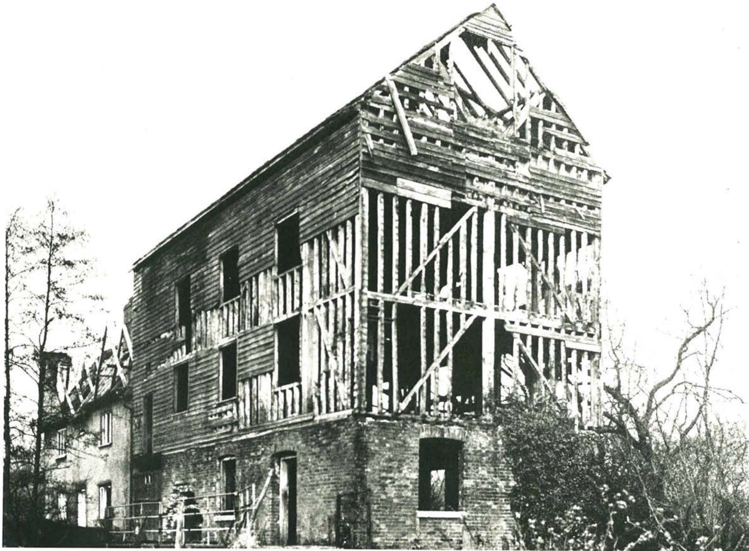
Early nineteenth century light stud framing in southeast England. (Mercer, Vernacular , after p. 122)
