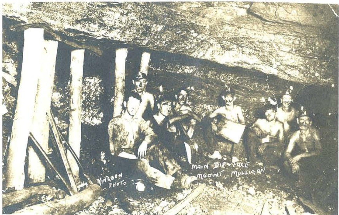
Miners in the underground workings about 1930. Note the universal adoption of electric headlamps, and the timber props and stone packwall at left. (Kingdon / Jim McColm)
