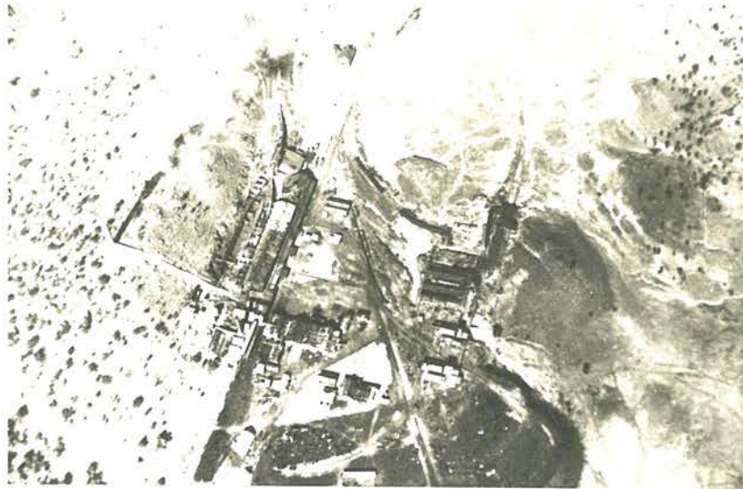
Chillagoe Smelters, 1934, aerial view looking west. (Oxley, Ball : Leica 13-18)
