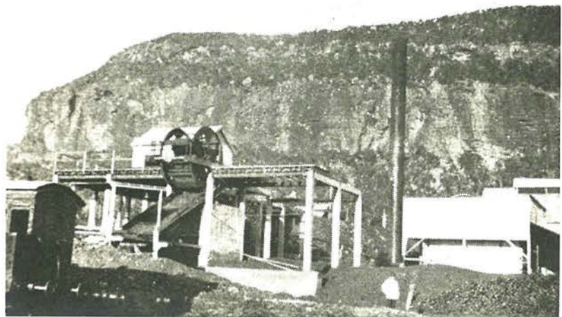
Tippler, coal screens and powerhouse, 1917, looking southwest. (Ball/Q.G.M.J. 15 October 1921, p.396)
