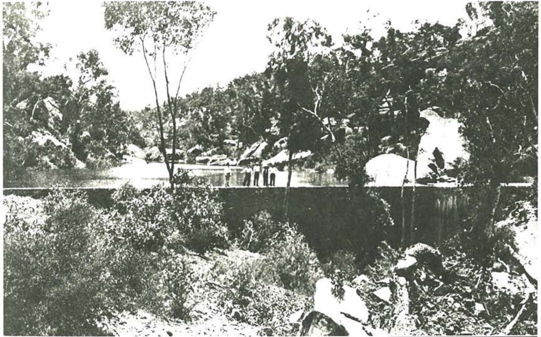
The dam on Richards Creek on top of the mountain, after raising, 1921, looking south. ( Q.G.M.J. 1922, frontispiece)
