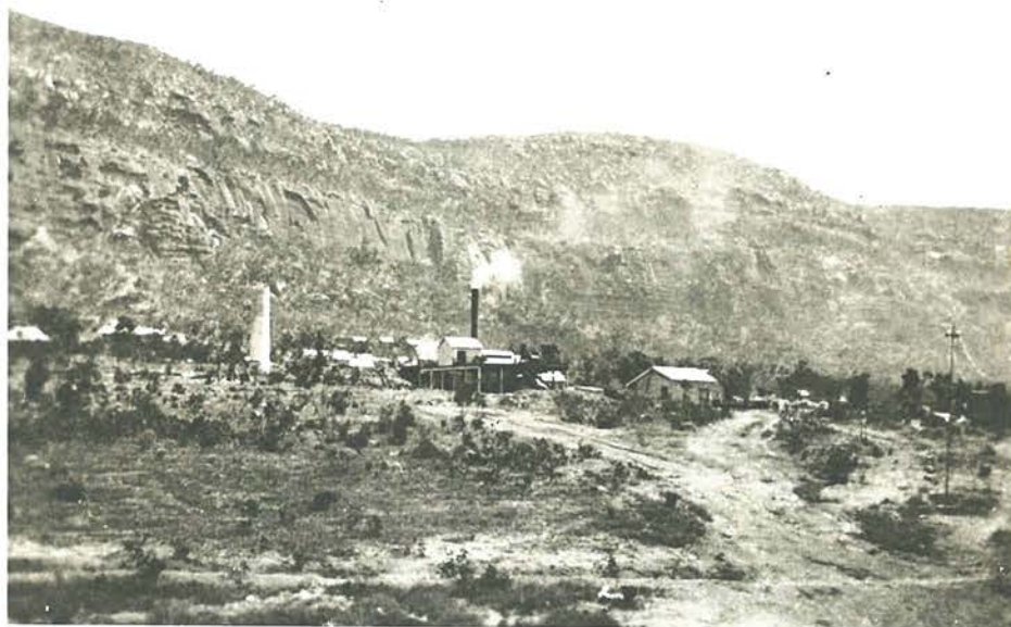
The mine surface workings from the town, 1920, looking northwest. The coal-loading tippler is in the centre, with the half-completed stack to the left. (Hynes/Elsie Kirkwood)
