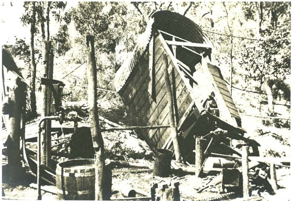
The wreckage of the switchboard and blacksmith's hut, near the mine entrance. (Taylor/ Q.G.M.J. 15 October 1921, p.399)
