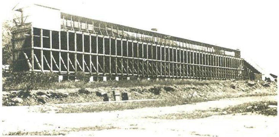
The coal bin and conveyer, 1925, looking northwest. ( Q.G.M.J. 15 June 1925, p.220)
