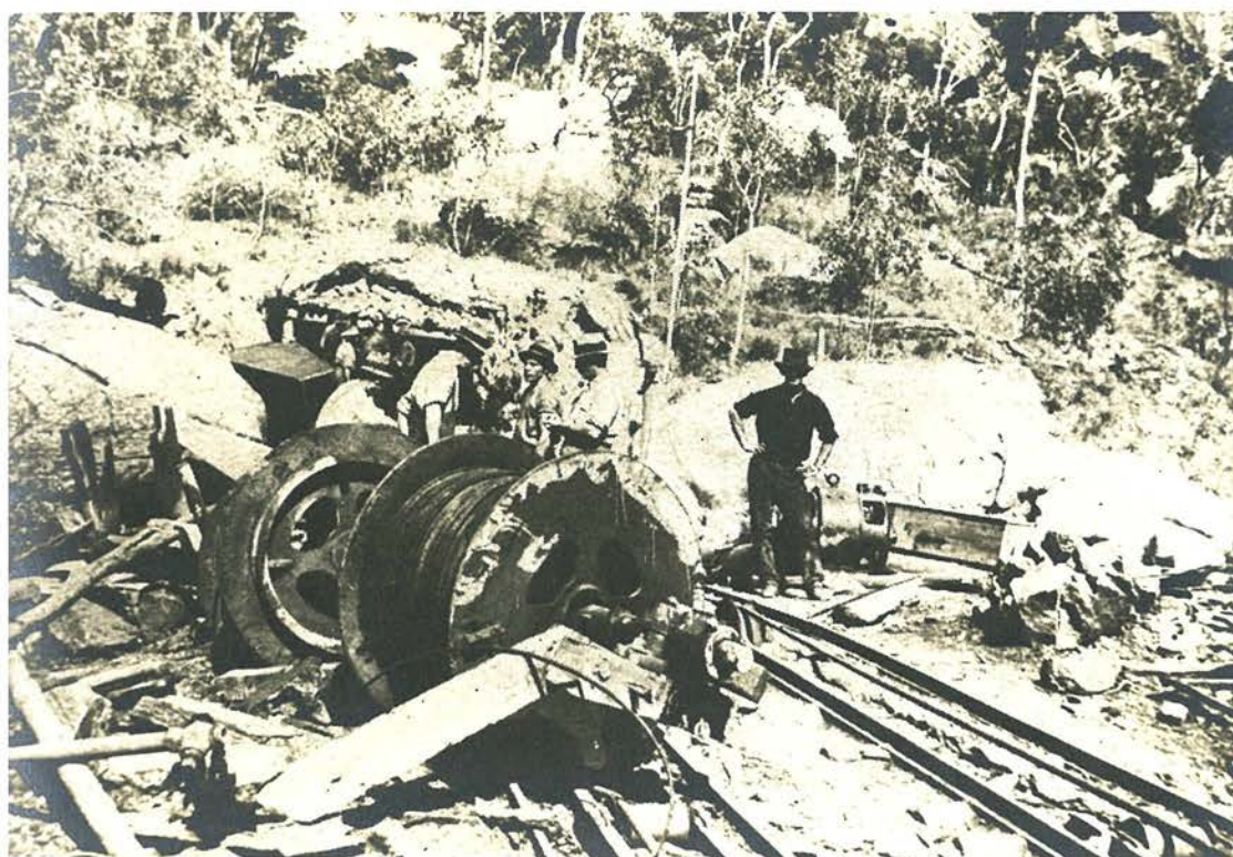
The steel cabledrums from above the mine entrance, blown twenty metres down the ropeway by the explosion. (Taylor/ Q.G.M.J. 15 October 1921, p.399)
