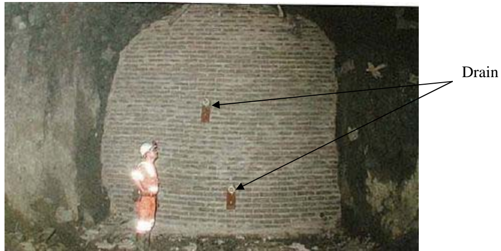
Figure 3.4 Example of barricade in a stope (After Potvin et al. 2005)
