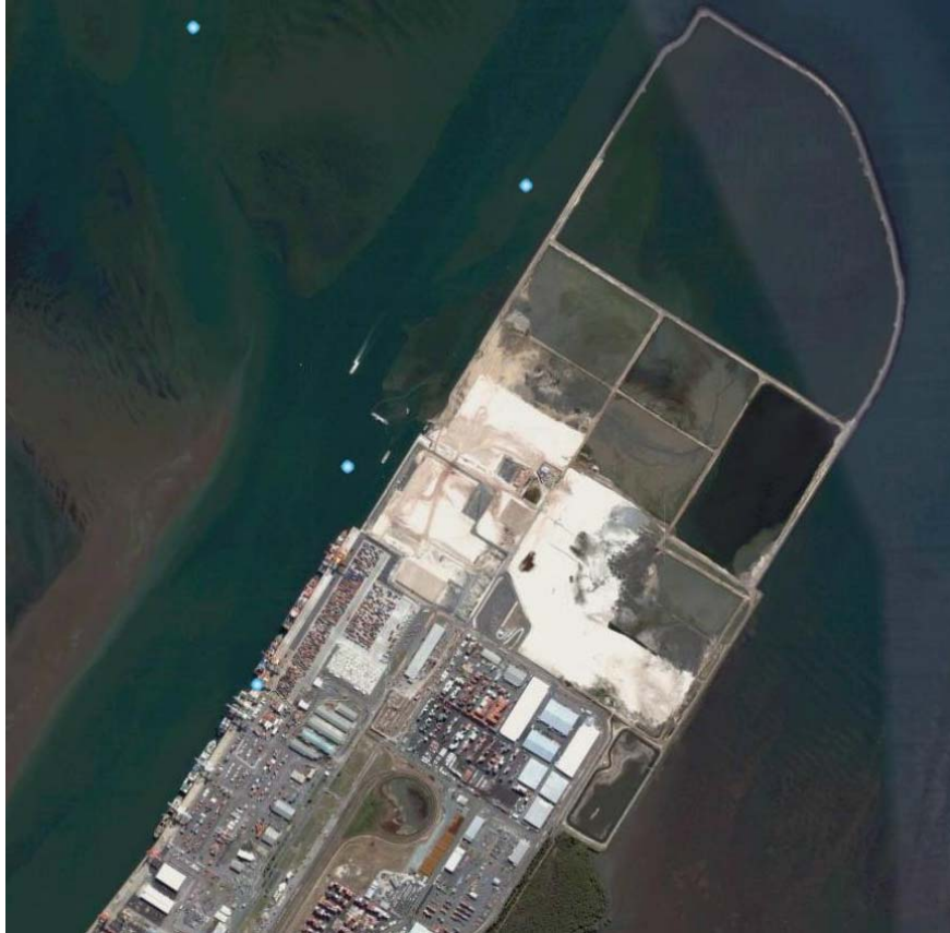
Figure 2.17 Aerial view of the Port of Brisbane
