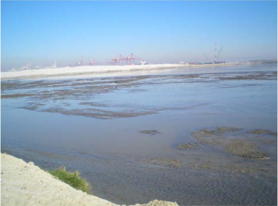
Figure 4.2 Paddock in the Port of Brisbane filled with dredged mud from Moreton Bay
