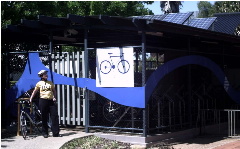
Study 7 Figure 7 Solar panels and green technology at the “end of trip facilities” for bicycle users
