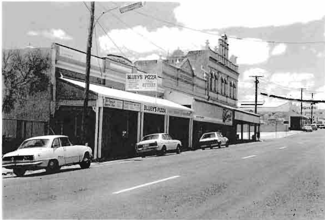
Figure 4.11 : East side of Mosman Street, to south from Elizabeth Street ; from left, Bright building, Foy building, Ross's Building (destroyed by fire 1992), Gill Street, vacant, Whitehead building and Smith building (now Arthur Tittley Centre) (1992)
