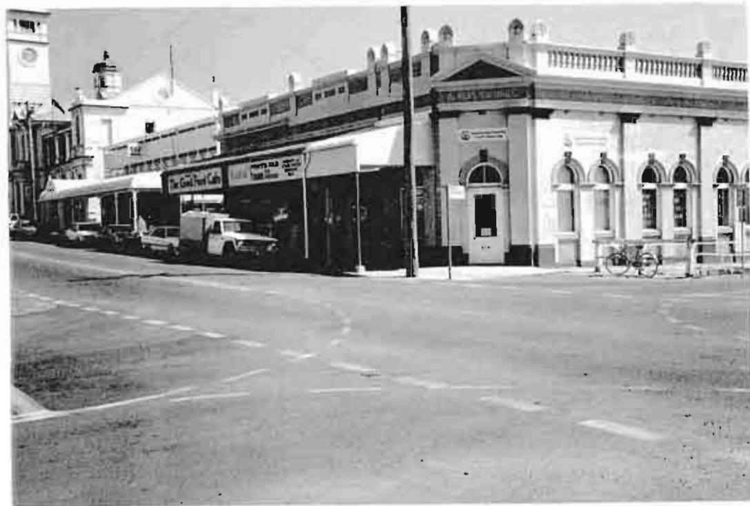
Figure 4.5 : north-west corner of Gill Street and Deane Street (1992) ; from left, Post office, Westpac Bank and Acker's Building
