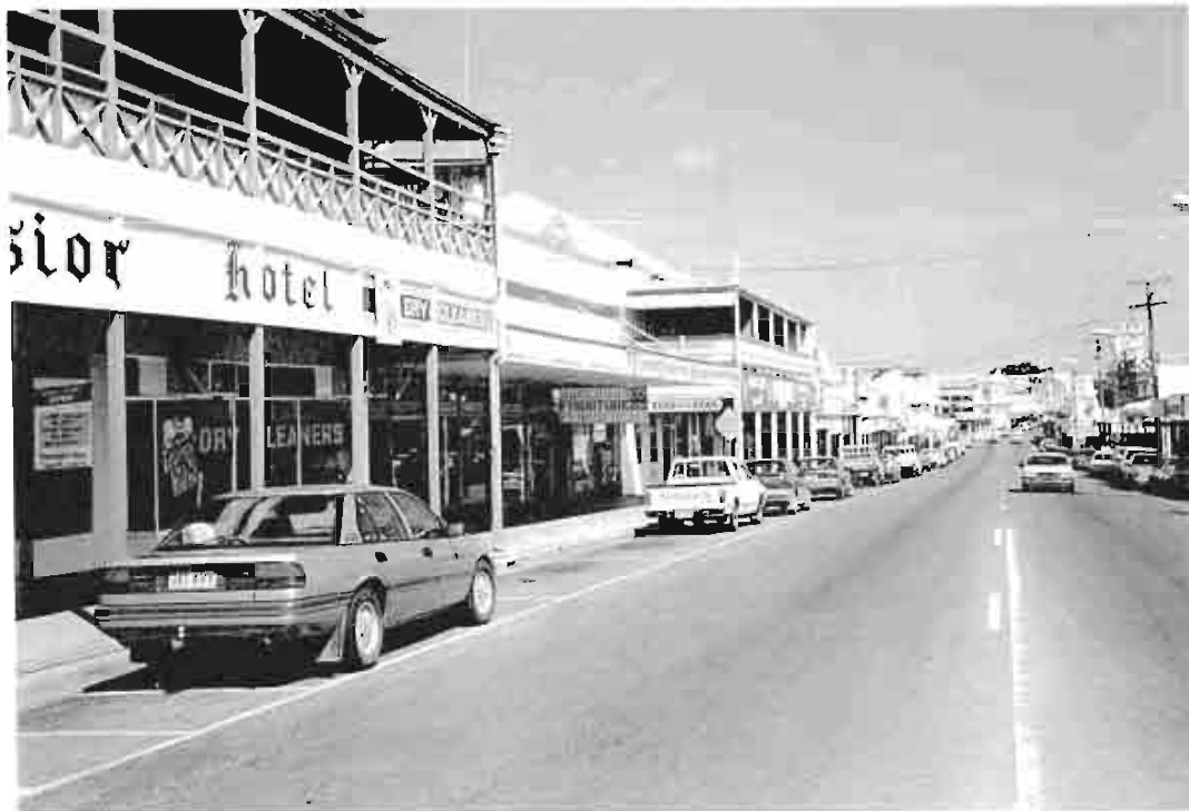
Figure 4.3 : Gill Street to west from Church Street. Excelsior Hotel on left. Court House Hotel with footpath verandah in centre. (1992)
