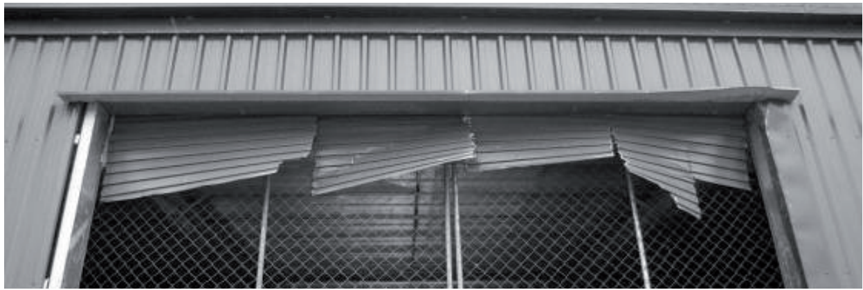
Figure 14: Torn sheet-type roller door.
