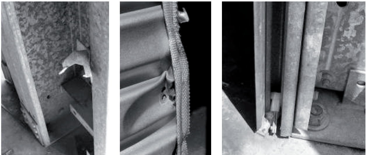
Figure 15: Failures associated with wind locks – (left) failed track bracket, (centre) wind lock torn from door and (right) wind lock in track.
