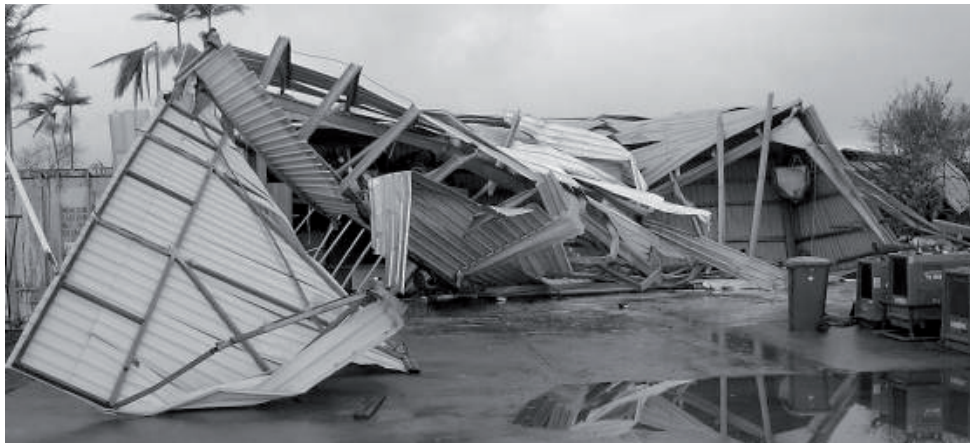
Figure 12: Collapse of cold-formed steel industrial shed.
