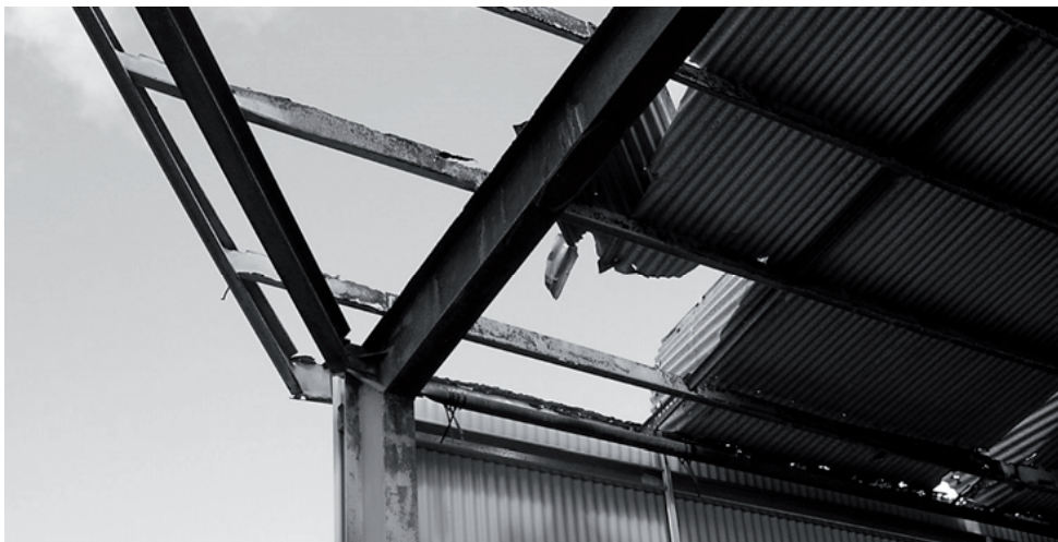
Figure 13: Hot rolled steel framed shed with severe corrosion of purlin.
