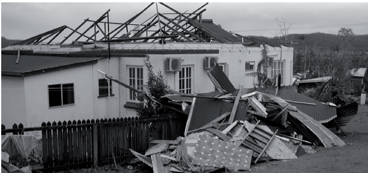
Figure 9: Loss of ridge beams.
