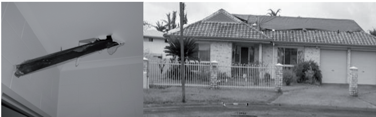
Figure 11: Debris damage to contemporary housing – (left) debris penetration through metal roof; (right) tile damage after debris impact.
