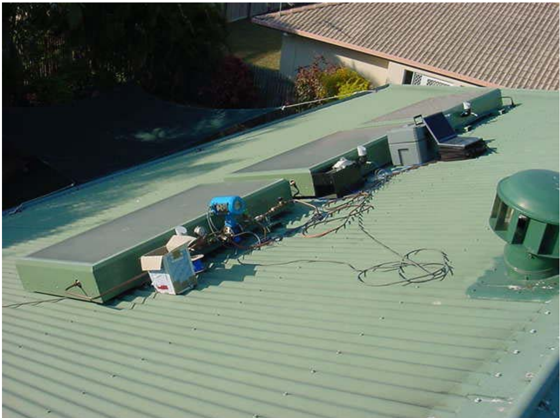
Figure 5.5. Experimental apparatus used to determine collector efficiency parameters
