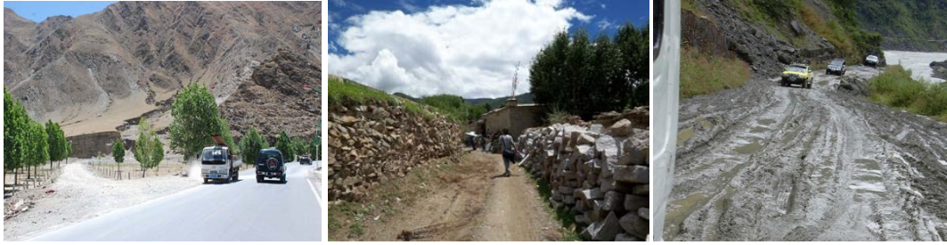
Figure 5. 9: The road situation in Caigongtang Town
