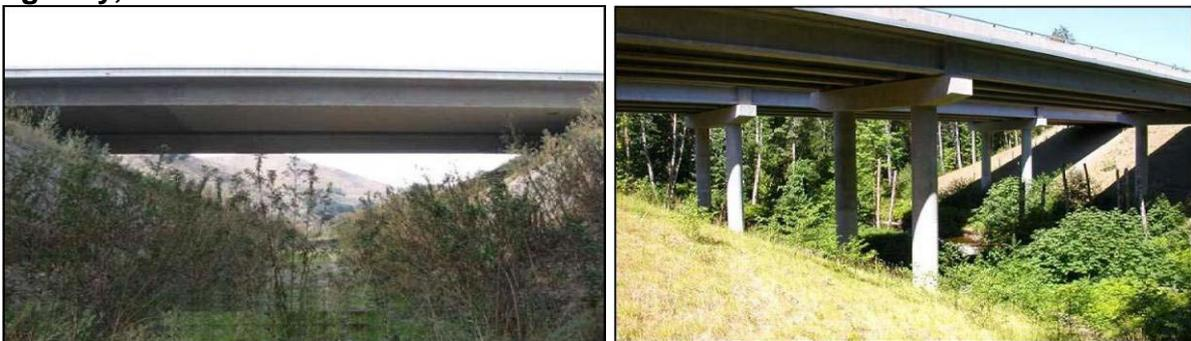
Photo: a) From Wildlife and Roads (2005). The original box culvert at this site was removed and a bridge installed to create an effective passage for bobcat and coyote. b) from Sielecki (2005)
