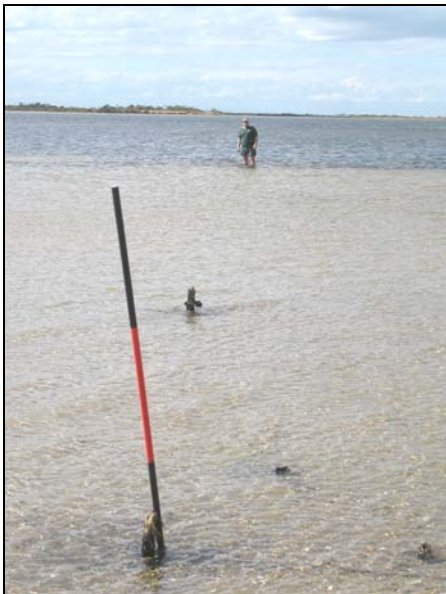
Figure B-2. 12: Duck Island pier piles which extend to the man in the distance.
