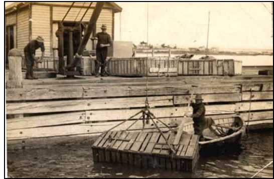
Figure 6. 7: Lowering a crayfish coff with the Fishermen's Pier Crane (Photo PH092, QHM Collection).
