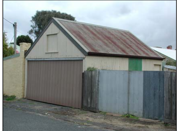
Figure 7. 47: Former morgue in Andrews St, Queenscliff.
