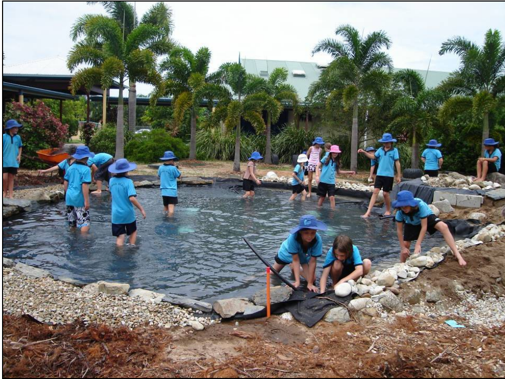
Plate 4.9. Constructing final stage of the mini wetlands at Whanilla SS
