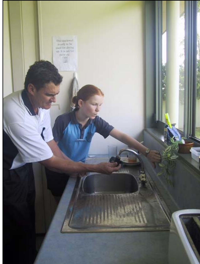
Plate 4.14. Fitting water saving devices at Hollindale SS
